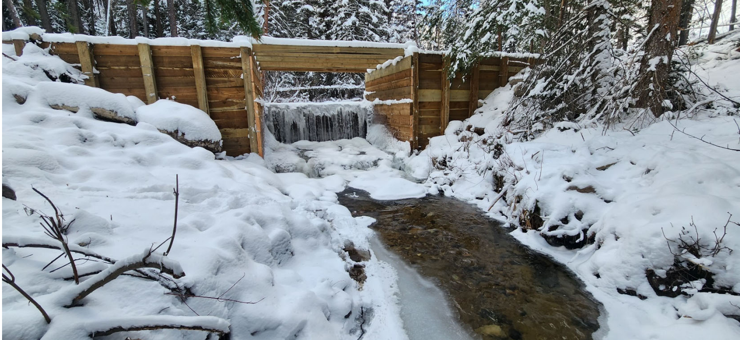
Figure 4. Example of wood crib fish barrier proposed for Dutchman Creek (Bryant Creek photo).
