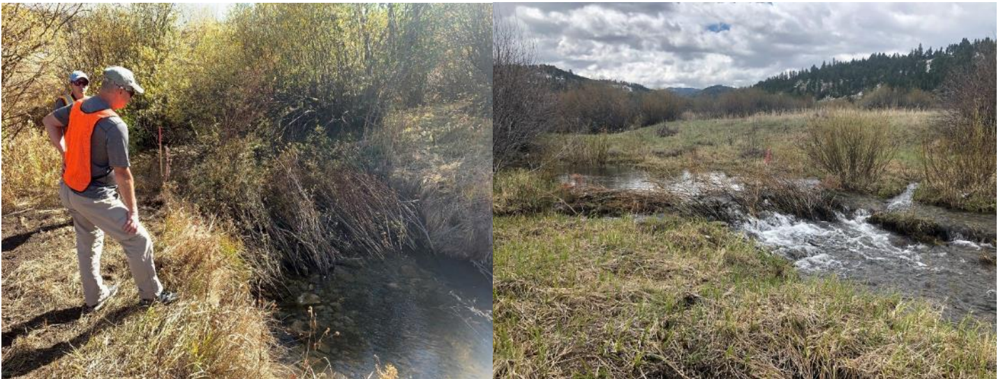
Figure 4. Example of Beaver Habitat Structures (BHS) installed in the main stem of Spotted Dog Creek. These structures are meant to mimic beaver dams but are created with coarse bed material so that they can survive multiple runoff pulses even in incised channels. The BHSs are designed to route flows out of the incised channel and onto the floodplain during high-water events and provide scaffolding from which beavers can build robust dam complexes that will lead to long-term recovery of the stream channel and floodplain. The left panel shows a BHS just after construction, where a mat of willows is placed on the structure to encourage adventitious root growth and attract beavers to the site. The right panel shows a BHS during a high flow event. BHSs are built in a series of 5-10 structures that all back up water to the next structure upstream. This arrangement mimics natural beaver dam complexes and provides structural redundancy in the stream channel so that the effectiveness and resiliency of these BHS complexes does not depend on any single structure.
