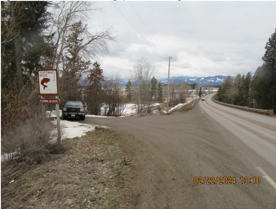
Figure 9. Approach to the existing Sportsman’s Bridge FAS
