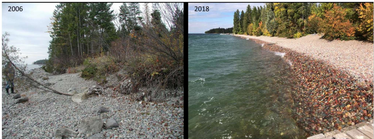
Figure 3. A September 2018 photograph looking north over the gravel beach fronting the CSKT campground at Blue Bay (right photo). This beach was constructed in 2007 and has functioned as a shore protection structure for over a decade now. It currently exists in a state of dynamic equilibrium where it adjusts and shifts in profile to summer storm waves while at the same time not washing away. It does this because wave action pushes gravel up the beach face forming a crest rather than washing it offshore (Lorang 2000, 2002). The waterline shows the height to which wave swash runs up the beach face. Before 2007 this shoreline was eroding with the lake level extending all the way to the vegetation line seen here at the top of the gravel beach (left photo). (Lorang 2023)
