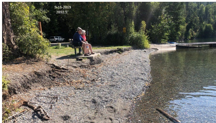
Figure 1. This photograph shows how narrow the remaining beach is at the boat launch when the lake is 6" below full pool (2893' Somers Datum). At full pool the beach disappears allowing waves to break directly against the bank. At lower lake levels breaking waves erode the bank and undermine the park bench and other infrastructure at the State Park. (Lorang 2023)
