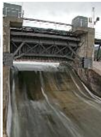
A RIVER FREED Clockwise from top left: Looking north, Milltown Dam in 2005 before removal at the confluence of the Blackfoot (center of photo, below the bridge) and the Clark Fork; the dam spillway that blocked fish movement for more than a century; the Clark Fork flowing free after the dam was removed in 2008-09; following sediment removal, rechannelling, and native vegetation planting, Milltown State Park now sits where the reservoir once was.
