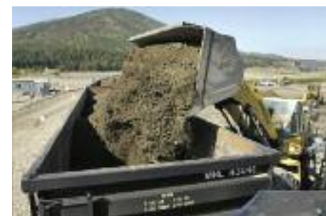
BAD DIRT Removing toxic sediment from below Milltown Reservoir after drainage.
