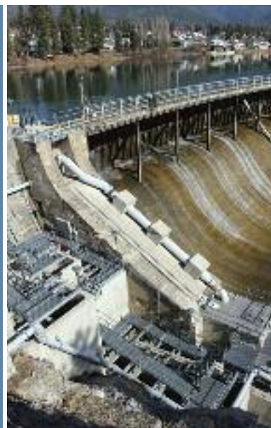
CLIMB, FISH, CLIMB Left: In 2015, a small fish ladder was installed to help spawning brown trout from Ennis Lake migrate into Smith Lake. Anglers reported seeing brown trout upstream of the ladder just a few months after installation. Right: Built in 2009, the $10 million Thompson Falls fish ladder is the first full-height fish passage in the United States constructed specifically for bull trout. After 95 years, the fish once again migrate upriver past Thompson Falls Dam into hundreds of miles of native spawning waters in the upper Clark Fork drainage.
