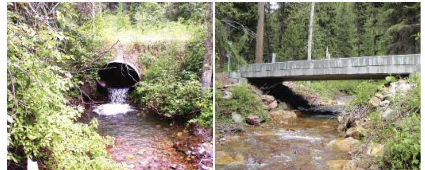
REMOVING SOME BARRIERS WHILE CREATING OTHERS Top left: A typical “perched” culvert on a tributary of the Blackfoot River blocked upstream bull trout and westslope cutthroat trout migration by creating a waterfall during low water and a high-velocity torrent during spring runoff. As in many forested watersheds across western Montana, the culvert was replaced by a free-span bridge (above right) that allows for natural fish movement. Below left: A natural waterfall on Ruby Creek near Ennis protects a reintroduced westslope cutthroat trout population upstream from hybridization by non-native rainbow trout below. Below right: FWP built this concrete box culvert on White Creek, a tributary to Canyon Ferry Reservoir, to safeguard pure-strain westslope cutthroat trout above the structure from non-native fish downstream.
