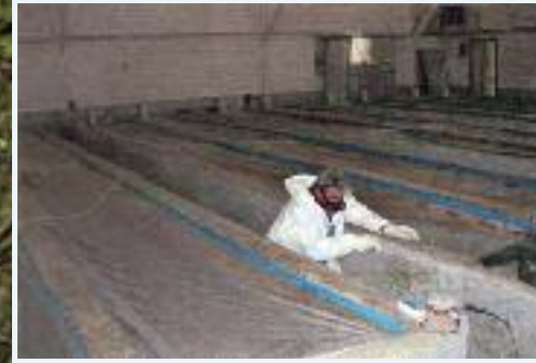
CLEANUP CREWS Once the Lewistown hatchery was determined as the PCB source, FWP contracted to have it and the creek downstream cleaned. Left: A notice warning anglers to release all fish on Big Spring Creek. Above: Crews removed all old paint and repainted contaminated raceways. Right: Vacuuming bottom sediment just downstream from the hatchery.
