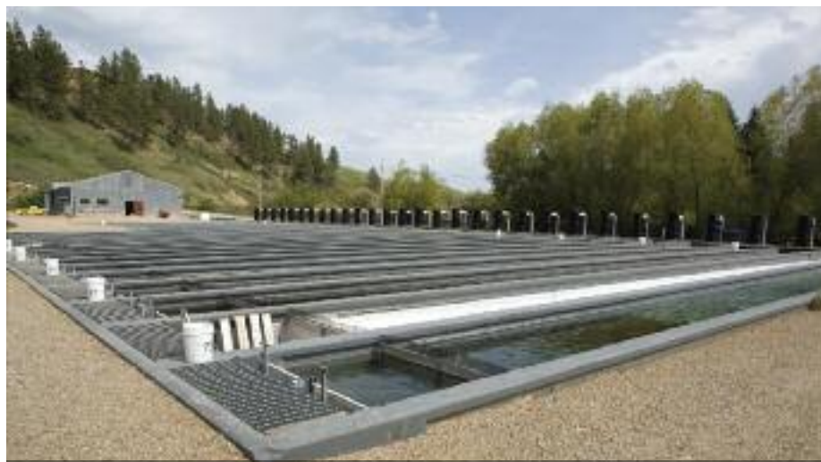
SILVER LINING One bright spot in the PCB contamination saga was that FWP's Big Springs Trout Hatchery was revamped with new raceways, tanks, and other features that allow it to produce fish more efficiently and cost-effectively.
