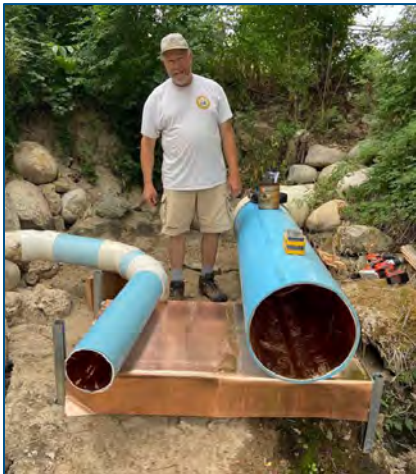
Figure 7. Dave Ellis stands next to biosecurity upgrades at FWP's Bluewater Fish Hatchery. Copper pipe lining prevent movement of macroinvertebrates, such as New Zealand mudsnails, into the hatchery as well as an extended effluent pipe that creates a higher drop to prevent animals from entering the pipe.
