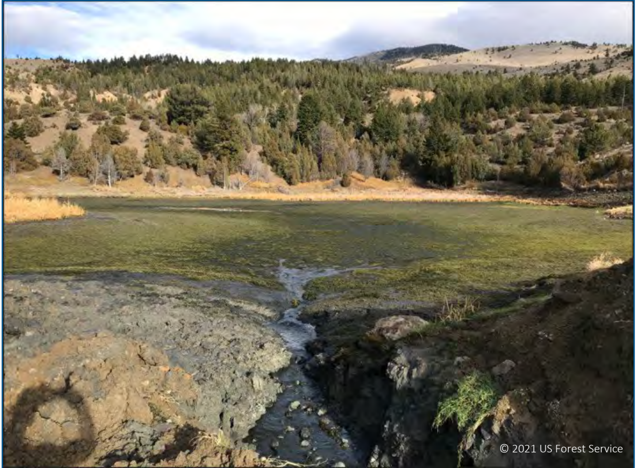
Figure 19. Middle Slip and Slide Creek Pond on USFS land near Gardiner, MT. It was drained in 2021 to remove the high-hazard dam status and to eradicate curlyleaf pondweed.
