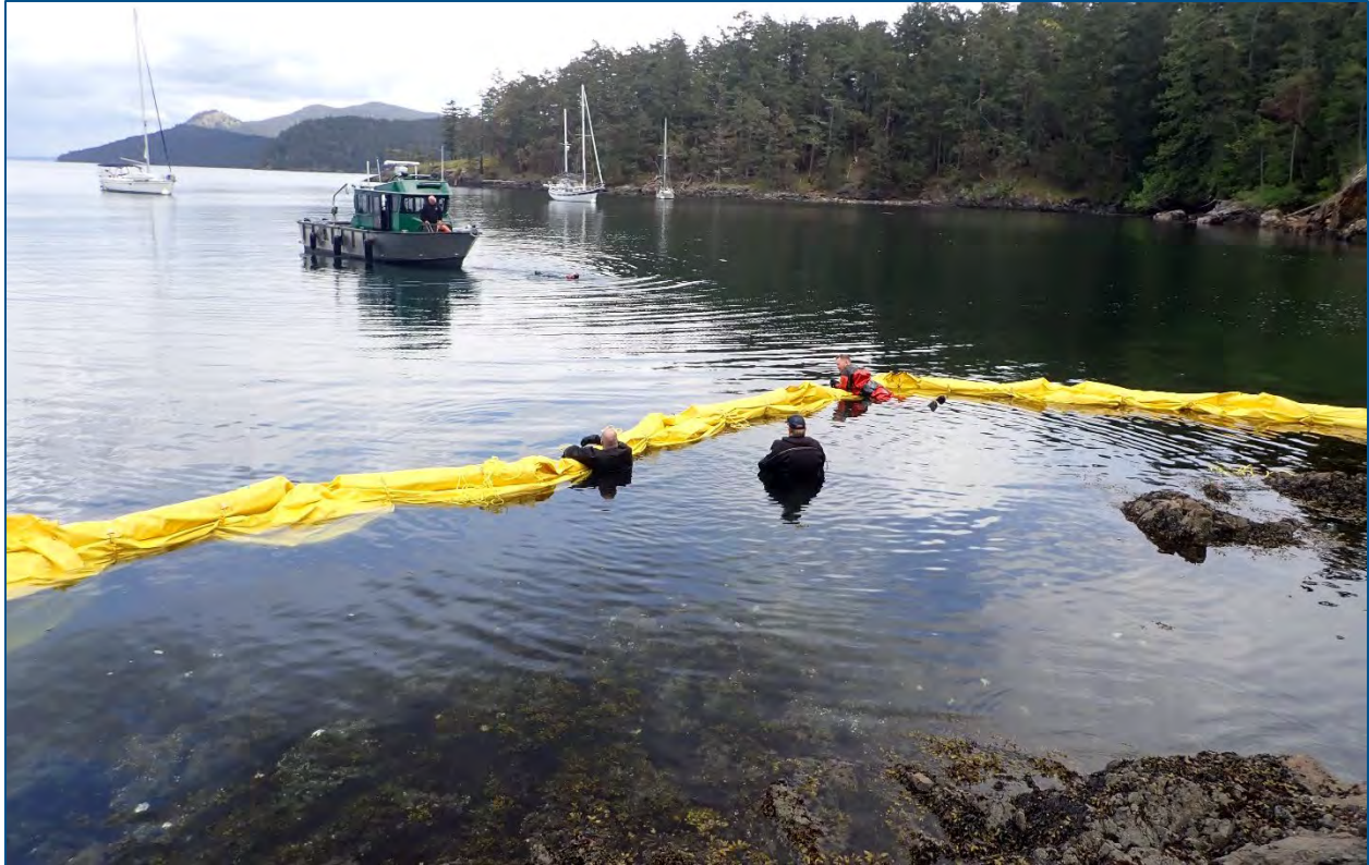
Figure 2. Shore support helps deploy the containment boom. A similar containment boom could be used in Montana in the event of a discovery of a dreissenid mussel population in order to contain and/or treat it.
