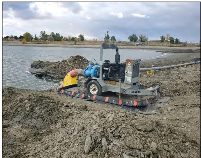
Figure 25. The pump used to dewater the remaining approximately four feet of water that remained after passively draining all possible water through the irrigation control structure.
