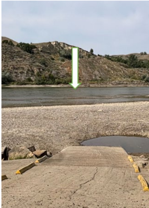
Figure 8: Roche Jaune FAS, Miles City (09/2025). Arrow indicates the location adequate water depth is present (>2') to float a boat off a trailer, 400 feet from the end of the boat ramp.
