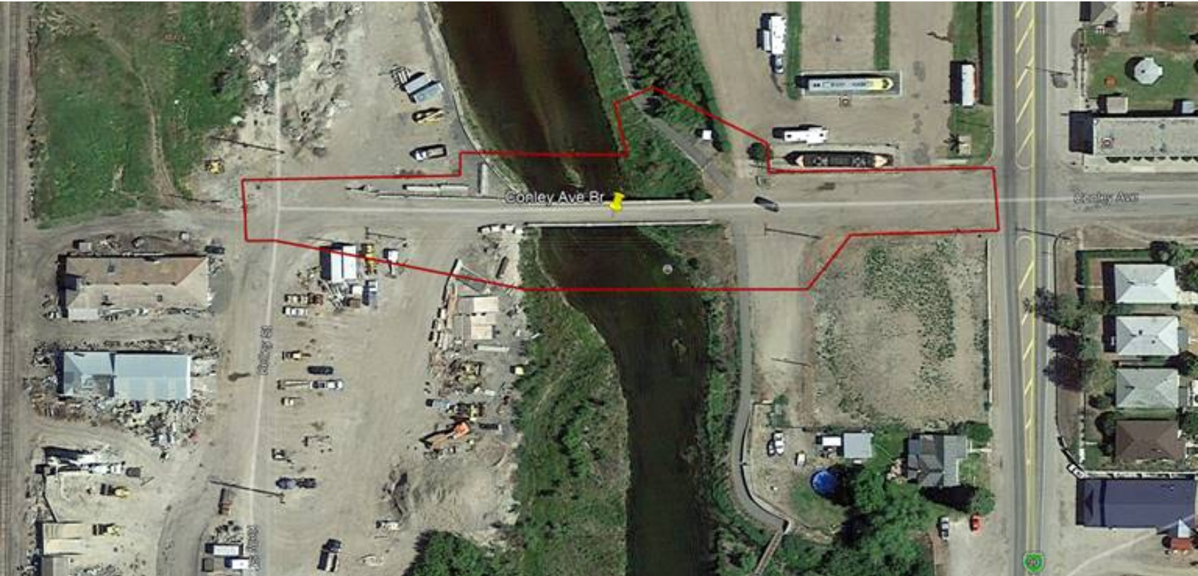
Aerial view of project area showing anticipated construction limits.
