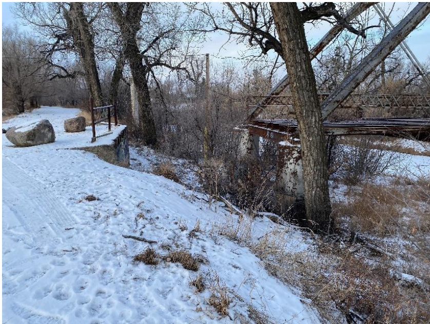
Profile view of existing approach span (south end shown).
