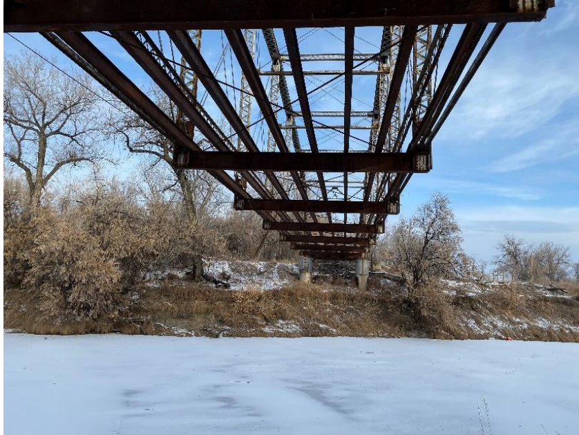
Underside view of bridge.
