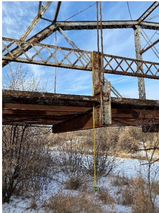
View of original lattice bridge rail.
