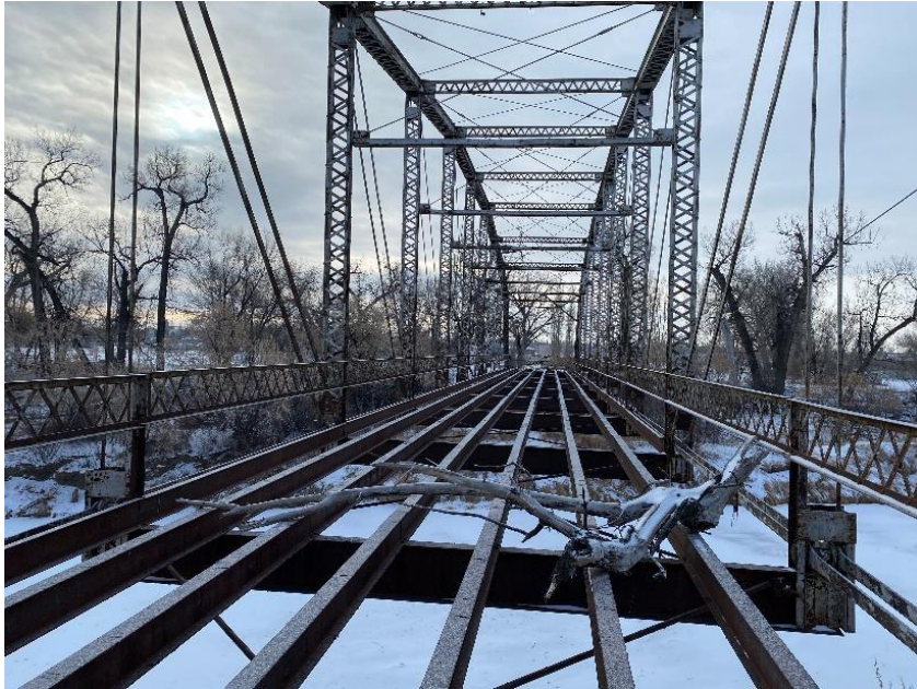
View of existing truss superstructure
