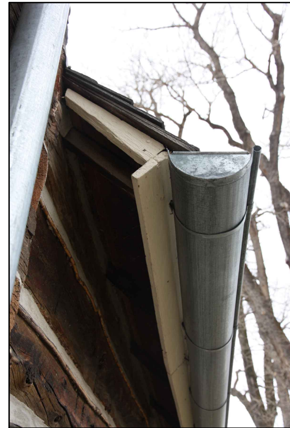
CHIEF'S HOUSE TYPICAL EAVE & GUTTER (NORTH)
