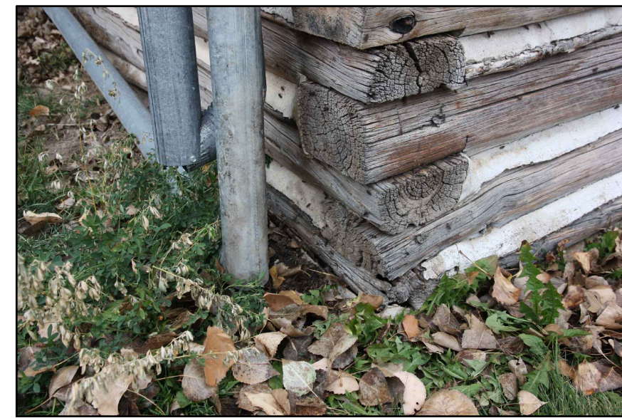
CHIEF'S HOUSE DOWNSPOUT AT SOUTHWEST CORNER
