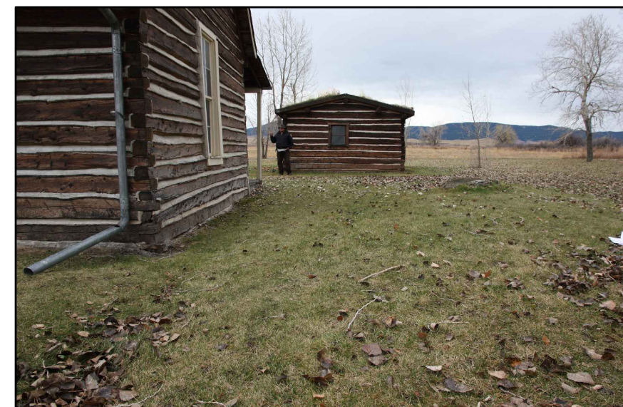
NORTHWEST CORNER, SHOWING EARTH SLOPING DOWN TOWARDS WEST SIDE ON BUILDINGS
