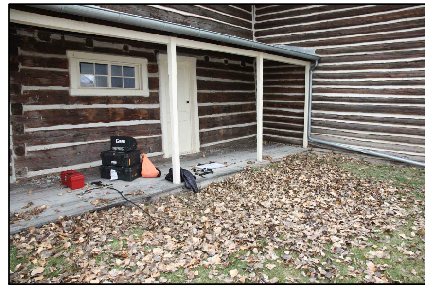
CHIEF'S HOUSE LEAVES PILED UP IN FRONT OF SOUTH PORCH
