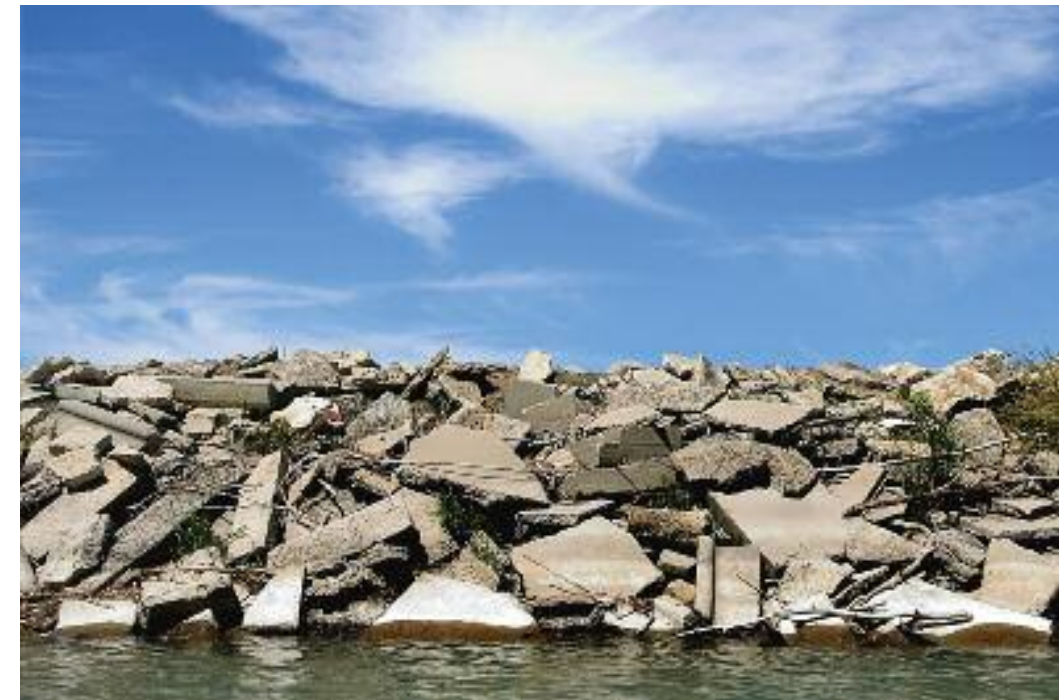
THE NEED TO MEANDER Above: When spring floods reconfigure river channels, old channels become ponds for waterfowl and furbearers, or fill in with gravel that creates important habitat for aquatic insects that feed fish. Below: When landowners try to tame river movement with riprap, channels feeding underground habitats are sealed off. River movement stops, and with it the natural flow of nutrients and water throughout the floodplain.
