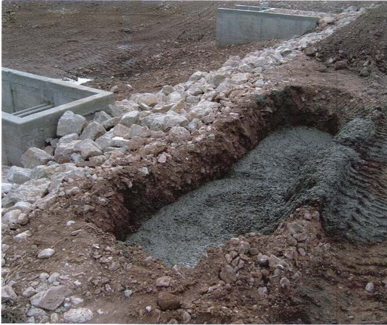
Figure 5: Bentonite plug installed to prevent leaking around the head gates.
