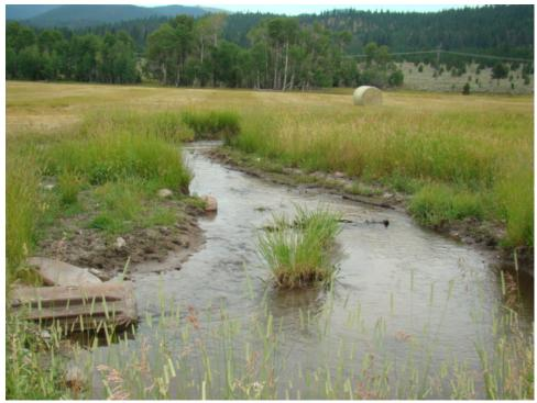
Upper crossing on Keep Cool Creek. This existing 2'x20' round culvert is proposed to be replaced with a 8'-1'' x 6'-1'' steel plate pipe-arch culvert.
