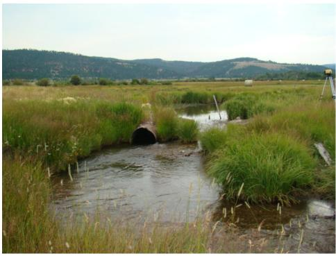
Existing lower crossing on Keep Cool Creek. This 2.5' by 20' long structure is proposed to be replaced with a hardened ford.
