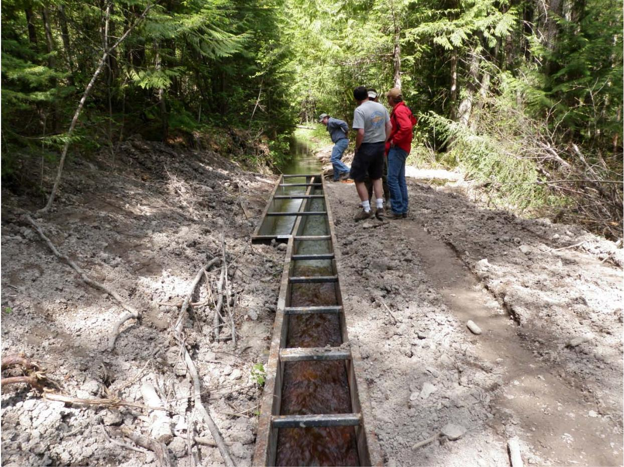
Figure 2. This photograph is a picture of an FCA Farmers fish screen that the Montana Chapter of Trout Unlimited installed on Sixmile Creek near Missoula, Montana. The proposed fish screen for the Deep Creek project would be similar.
