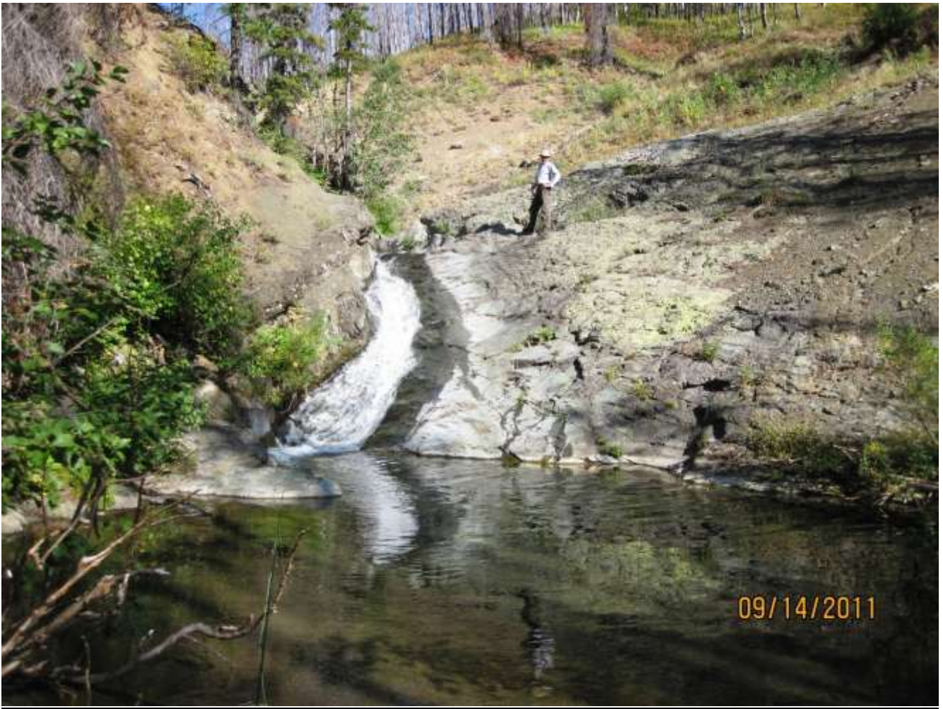
Figure 1. Fish barrier on Woods Creek.
