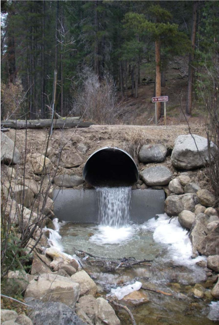
Figure 1. Fish barrier constructed at the Forest Service Road Crossing on the North Fork of Doolittle Creek
