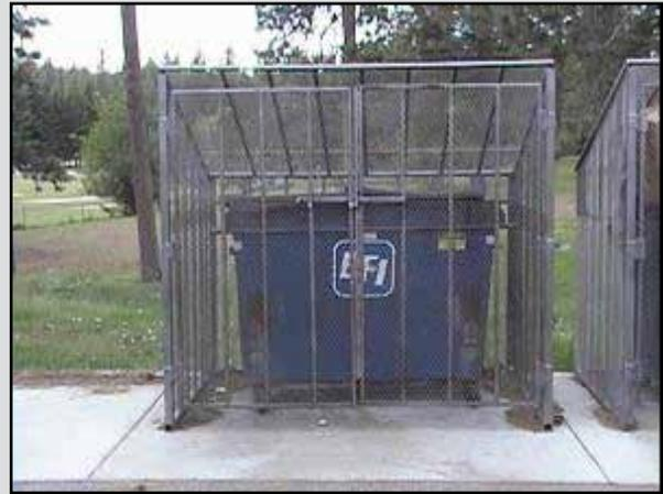
*Figure C.4-3. Illustrations of (A)-type Bear-Resistant Enclosures*
