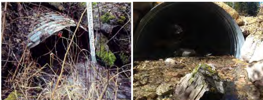
FIGURE 8. MARSHALL CREEK FISH PASSAGE BEFORE (L) AND AFTER (R).
