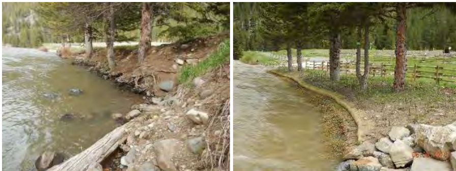
FIGURE 18. MOOSE CREEK GALLATIN RESTORATION BEFORE (L) AND AFTER (R) CONSTRUCTION.
