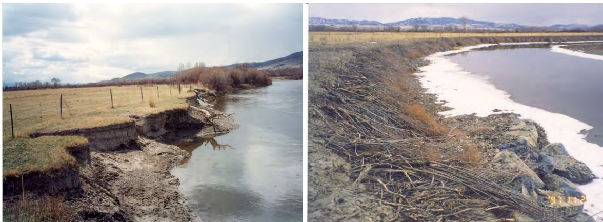
FIGURE 139. MISSOURI RIVER SIDE CHANNEL BEFORE CONSTRUCTION (L, 1996) AND AFTER CONSTRUCTION (1997, R).
