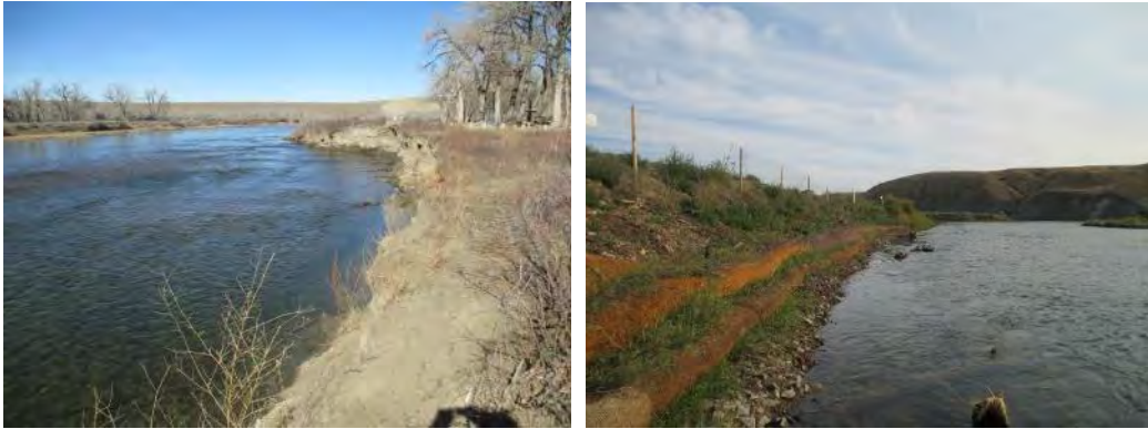
FIGURE 29. MARIAS RIVER BEFORE (L) AND AFTER (R) CONSTRUCTION.
