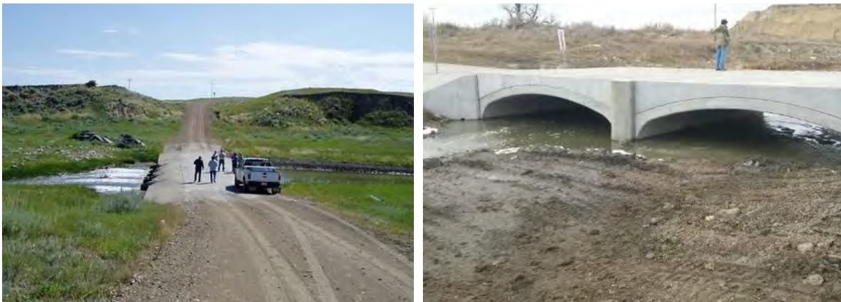
FIGURE 34. REDWATER RIVER BEFORE (L) AND AFTER (R) CULVERT REPLACEMENT.
