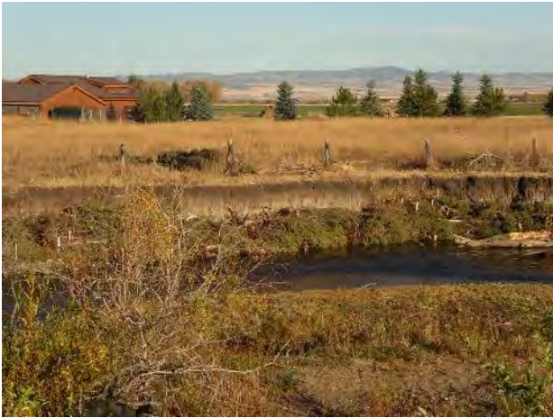
FIGURE 50. JUNIPER REVETMENTS CABLED INTO BANK 3.
