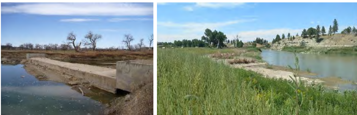
FIGURE 32. PRE-PROJECT FLANKED DIVERSION (L) AND POST PROJECT RESTORATION (R) ON THE MUSSELSHELL RIVER.
