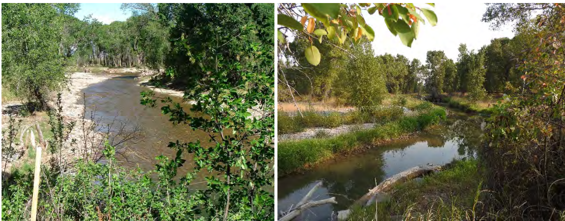
FIGURE 131. ELK CREEK CHANNEL RESTORATION, AFTER COMPLETION (L) AND IN 2017 (R).
