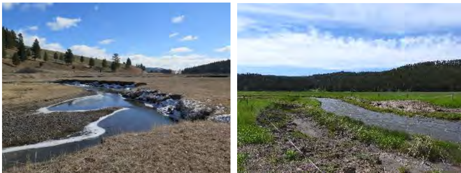
FIGURE 10. NEVADA CREEK CHANNEL RESTORATION BEFORE (L) AND AFTER (R).
