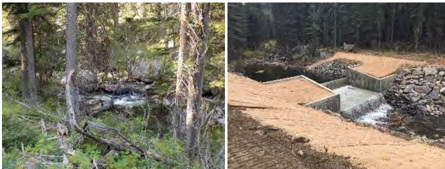
FIGURE 19. NORTH FORK SPANISH CREEK BARRIER BEFORE (L) AND AFTER (R) CONSTRUCTION.
