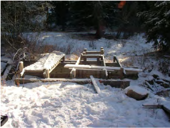
FIGURE 71. PIN AND PLANK IRRIGATION DIVERSION ON NORTH FORK HORSE CREEK.
