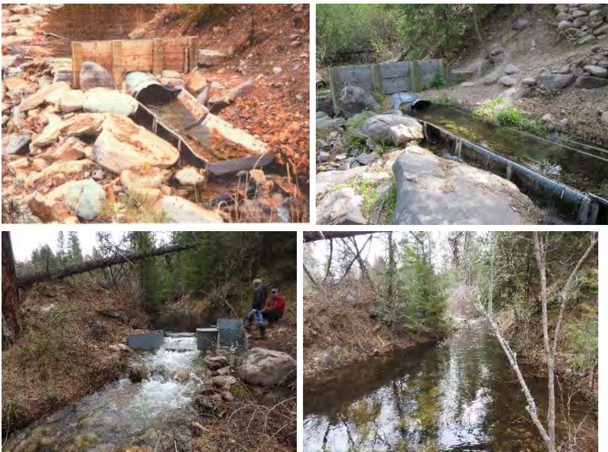
FIGURE 33. RATTLESNAKE CREEK BEFORE (BRENCAIL-TYPE SCREEN, TOP) AND AFTER (COANDA-TYPE SCREEN, BOTTOM).
