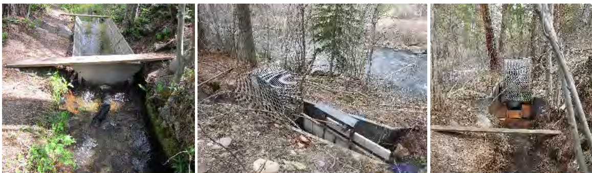
FIGURE 15. RATTLESNAKE CREEK COBBAN FISH SCREEN BEFORE (L), AND AFTER (CENTER AND R).
