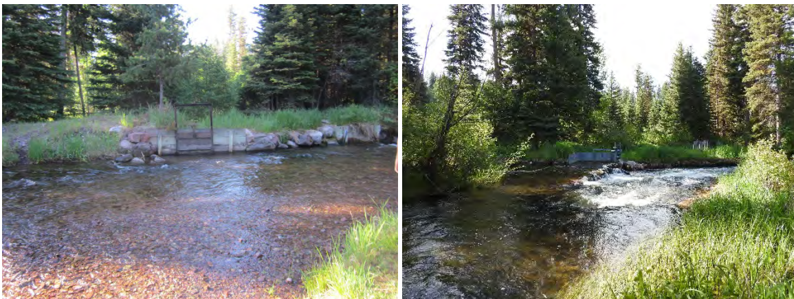
FIGURE 148. TRAIL CREEK BEFORE (L) AND AFTER (2018; R) CONSTRUCTION.
