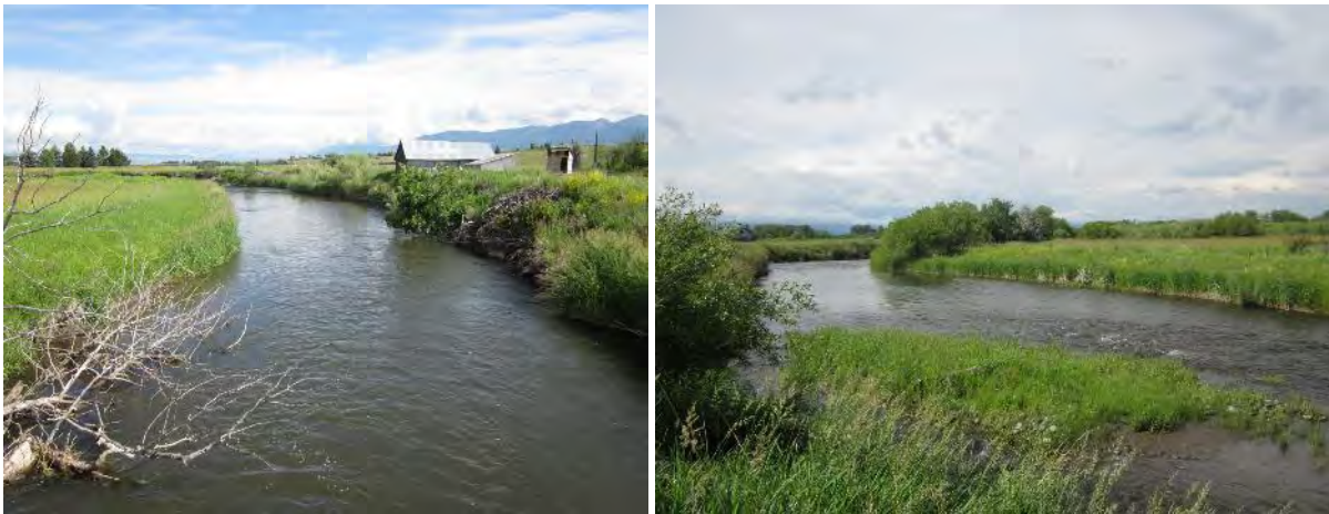
FIGURE 52. BANK 1 ON THE EAST GALLATIN RIVER BANK RESTORATION PROJECT, VIEWED FROM DOWNSTREAM (L) AND REESTABLISHED GRAVEL BAR NEAR BANK 1 (R).
