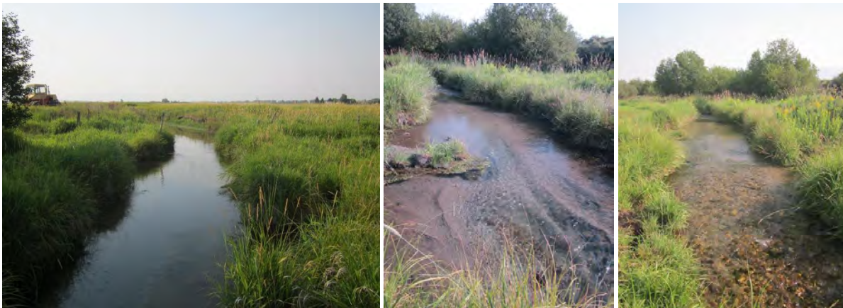
FIGURE 105. OVERLY WIDE CHANNEL (L), ACCUMULATION OF FINE SEDIMENT (C), AND EXPOSED GRAVEL (R) ON RESTORED PORTION OF SOUTH FORK ROSS CREEK.
