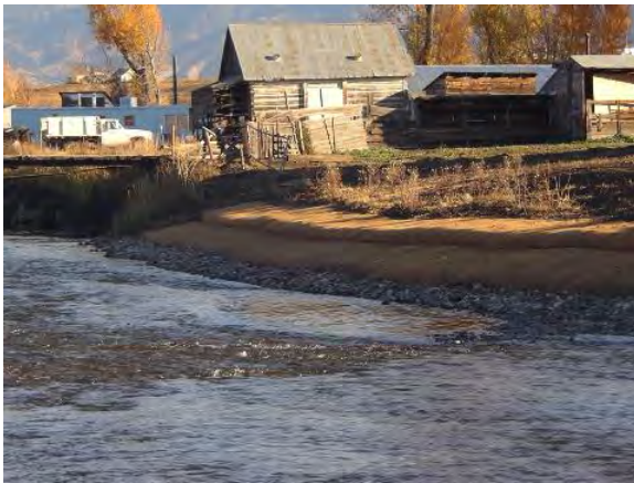
FIGURE 49. EXAMPLE OF FABRIC-ENCAPSULATED SOIL LIFTS ON BANK 2.
