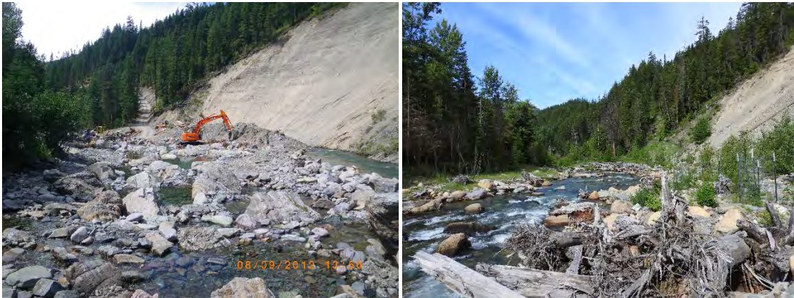
FIGURE 149. VERMILLION RIVER CHAPEL SLIDE STABILIZATION BEFORE (L) AND AFTER (2018; R).
