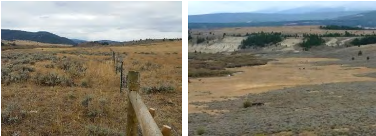
FIGURE 26. FRENCH CREEK RIPARIAN FENCING POST CONSTRUCTION.
