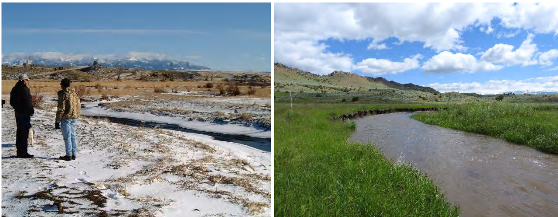
FIGURE 120. BRACKETT CREEK AFTER PROJECT CONSTRUCTION (L) AND IN 2017 (R).
