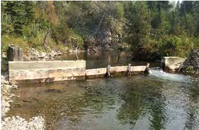
FIGURE 43. IRRIGATION DIVERSION ON COTTONWOOD CREEK.
