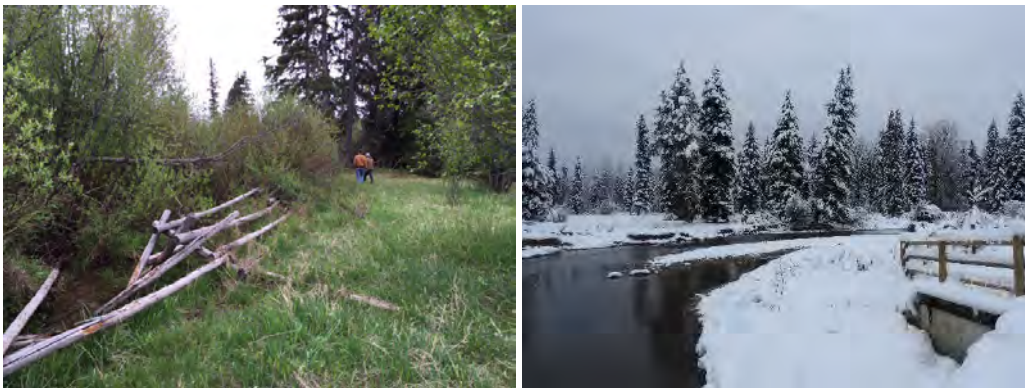
FIGURE 31. FAILING JACKLEG FENCE (L) AND NEW FENCE (R) ON MONTURE AND DUNHAM CREEKS.
