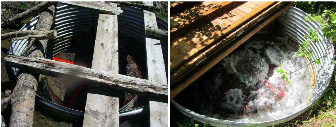
FIGURE 75. TURBULENT FOUNTAIN SCREEN WHEN NOT IN USE (L) AND IN USE (R) ON NORTH FORK HORSE CREEK.
