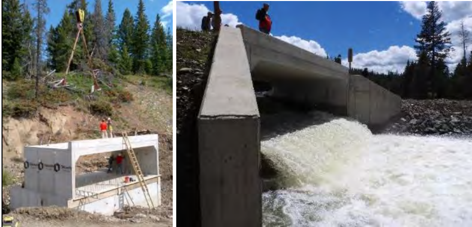
FIGURE 36. SHIELDS RIVER FISH BARRIER DURING CONSTRUCTION (L) AND AFTER INSTALLATION (R).
