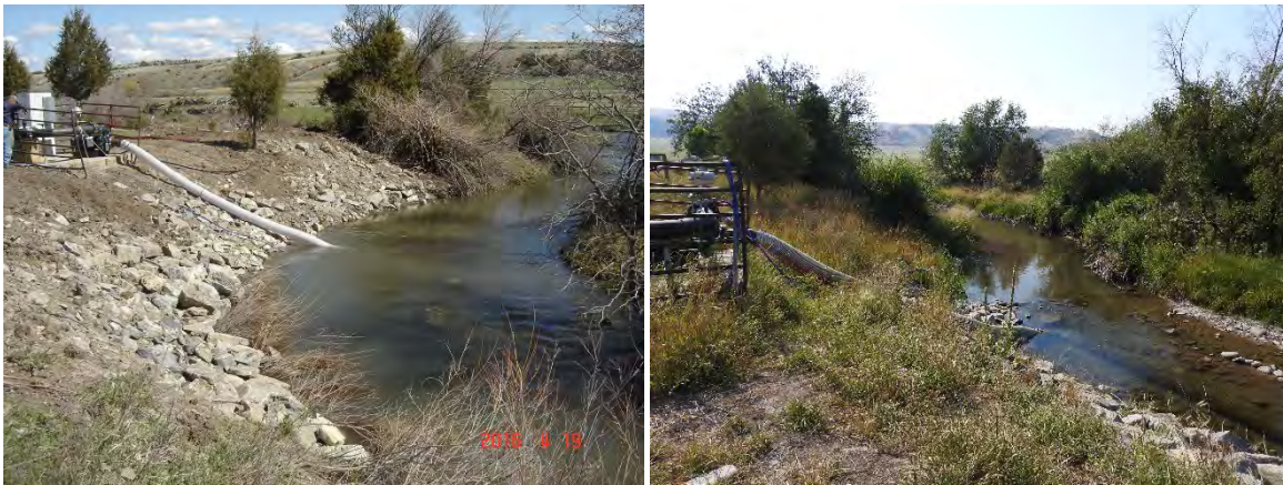
FIGURE 127. DEEP CREEK PUMP SITE AT COMPLETION (L) AND IN 2017 (R).
