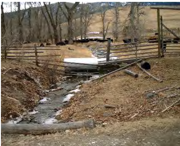
FIGURE 55. VIEW OF THE SPRING CREEK BEFORE PROJECT IMPLEMENTATION.
