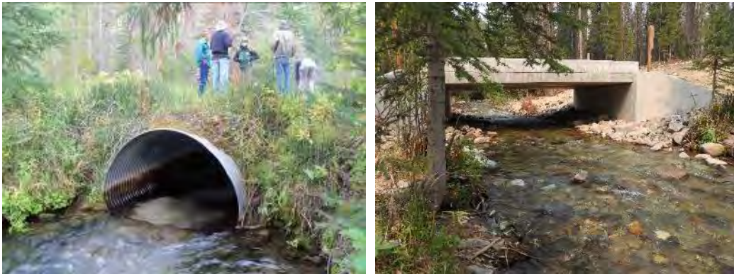
FIGURE 39. WARM SPRINGS CREEK BEFORE (L) AND AFTER (R) CONSTRUCTION.
