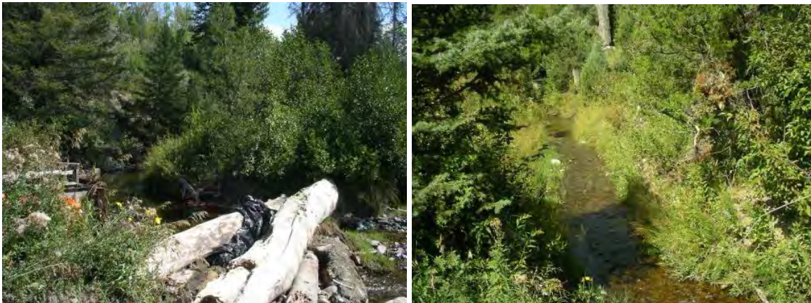
FIGURE 42. LOGS CHECKING COTTONWOOD CREEK'S FLOWS TO DELIVER WATER TO THE PIN-AND-PLANK HEAD GATE (L). WATER LEAKING INTO DITCH WHEN CHECK BOARDS WERE BLOCKING FLOW (R).
