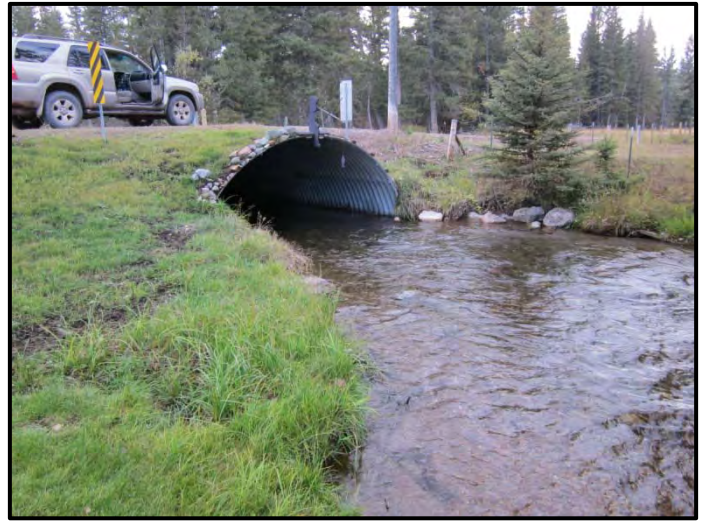
Photo Illustration 4. Fish passage enhancement projects completed at road crossings to allow for upstream migration. The upper two photos display a fish passage enhancement project located on Beaver Creek near the city of Havre in Hill County. The project replaced an undersized and perched culvert (photo on left) with an appropriately sized culvert set below stream grade. Beaver Creek supports rainbow trout, sauger and numerous species of native non-game fish. The lower two photos display a fish passage enhancement project located on Lincoln Spring Creek, a tributary to the Blackfoot River near the town of Lincoln in Lewis and Clark County. The project replaced an undersized and perched culvert (lower left photo) with an appropriately sized bottomless arch pipe (lower right photo). Lincoln Spring Creek supports brown trout, westslope cutthroat trout and potentially bull trout. The lower left photo was provided courtesy of Ryen Nuedecker, Big Blackfoot Chapter of Trout Unlimited.
