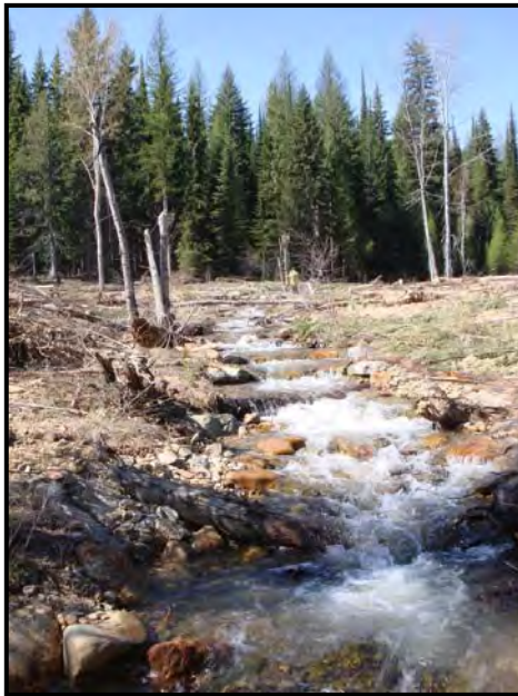
Photo Illustration 6. The reclamation of Mattie V Creek, a tributary to Ninemile Creek located in Missoula County that had been historically degraded by placer mining. Mine waste first had to be removed and re-graded starting in July 2010 (upper left photo). New channel construction was completed in August 2010 (upper right photo). The lower left photo shows the newly constructed channel undergoing its first spring run-off in May 2011. The lower right photo shows the re-vegetated stream banks and floodplain coming to life in August 2012. Mattie V Creek supports westslope cutthroat trout. The upper two photos and the lower left photo were provided courtesy of Rob Roberts, Trout Unlimited.
