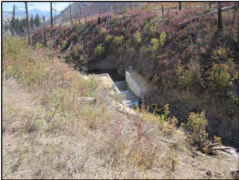
Photo Illustration 5. Fish passage barriers installed on two streams to protect the genetic integrity of native cutthroat trout from invasion by non-native rainbow trout. The upper photo shows a fish passage barrier installed on Lower Deer Creek, a tributary to the Yellowstone River located near the town of Big Timber in Sweet Grass County. Lower Deer Creek supports genetically pure Yellowstone cutthroat trout. The lower photo shows a fish passage barrier installed on Elkhorn Creek, a tributary to Holter Reservoir in Lewis and Clark County. Elkhorn Creek supports genetically pure westslope cutthroat trout.
