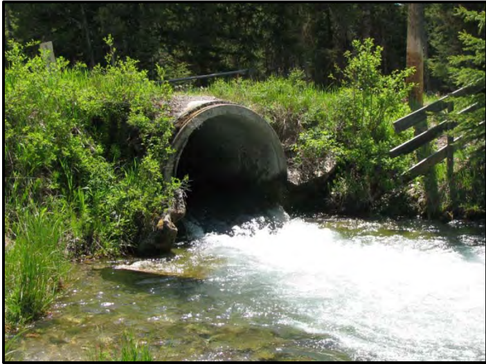
Photo Illustration 4. Fish passage enhancement projects completed at road crossings to allow for upstream migration. The upper two photos display a fish passage enhancement project located on Beaver Creek near the city of Havre in Hill County. The project replaced an undersized and perched culvert (photo on left) with an appropriately sized culvert set below stream grade. Beaver Creek supports rainbow trout, sauger and numerous species of native non-game fish. The lower two photos display a fish passage enhancement project located on Lincoln Spring Creek, a tributary to the Blackfoot River near the town of Lincoln in Lewis and Clark County. The project replaced an undersized and perched culvert (lower left photo) with an appropriately sized bottomless arch pipe (lower right photo). Lincoln Spring Creek supports brown trout, westslope cutthroat trout and potentially bull trout. The lower left photo was provided courtesy of Ryen Nuedecker, Big Blackfoot Chapter of Trout Unlimited.
