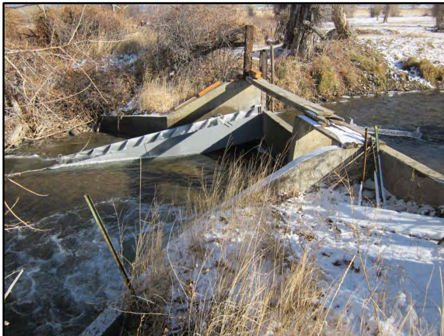
Photo Illustration 8. Fish ladders installed on two streams to improve upstream fish passage. The upper photo displays a fish ladder located on Frazier Creek, a tributary to the Blackfoot River located near Ovando in Powell County. Frazier Creek supports genetically pure westslope cutthroat trout. The lower photo shows a fish ladder installed on Prickly Pear Creek, a tributary to Hauser Reservoir located near East Helena in Lewis and Clark County. Prickly Pear Creek supports brown trout, rainbow trout and mountain whitefish.
