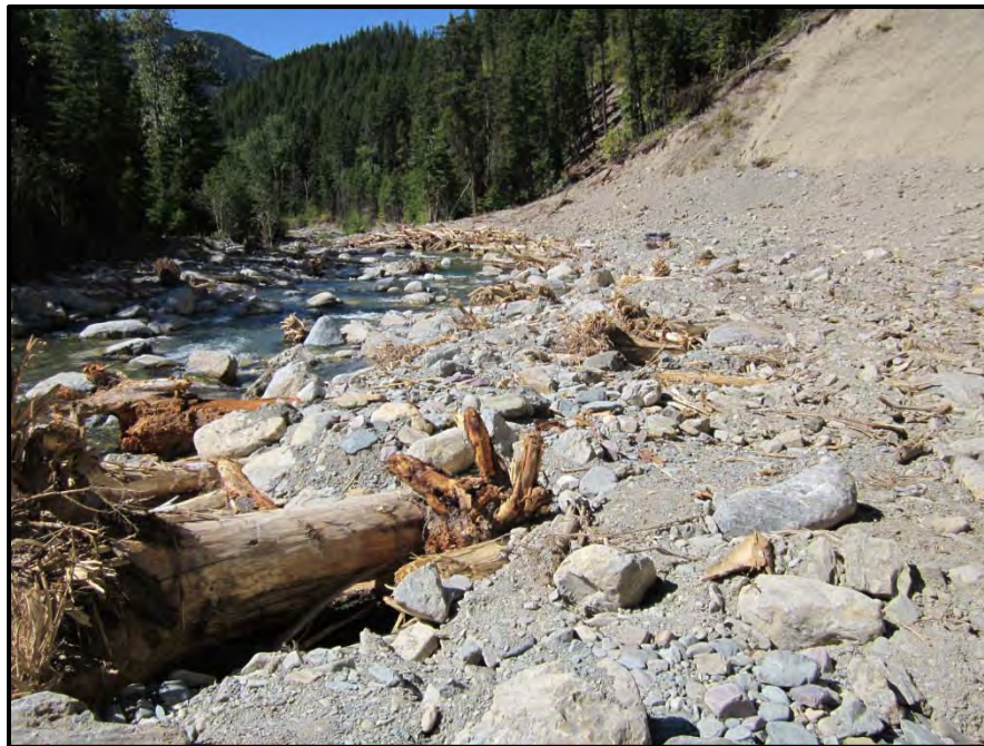
Photo Illustration 7. Stabilization of the Chapel Slide located on the Vermilion River, a tributary to the Clark Fork River in Sanders County. The upper left photo shows Chapel slide in 2009 prior to restoration. Stabilization involved moving the river channel away from the existing slide and constructing a floodplain bench at the toe (upper right photo). The lower photo shows the completed newly constructed river channel and associated floodplain bench in September 2012. The Vermilion River supports native bull trout, westslope cutthroat trout and mountain whitefish. The stream also supports non-native brown trout and brook trout. The upper two photos were provided courtesy of Craig Nesvig, Cabinet Ranger District.
