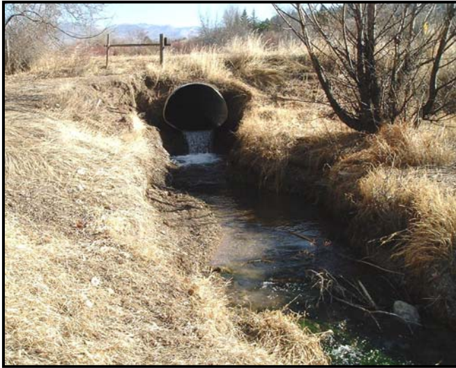
Photo Illustration 1. Upper two photos display a fish passage improvement project on Duck Creek, a tributary to Hebgen Lake. The goal of this project was to improve upstream fish passage, primarily for spawning rainbow trout from Hebgen Lake, through a culvert located on U.S. Highway 191. Photo on left shows perched culvert before project completion. Photo on right shows completion of constructed riffle downstream of culvert. Lower two photos display a fish passage improvement project on Magpie Creek, a tributary to Canyon Ferry Reservoir. The goal of the project was to improve upstream fish passage, primarily for spawning rainbow trout from Canyon Ferry Reservoir, through a culvert located on a U.S. Bureau of Reclamation road. Photo on left shows perched culvert before project completion. Photo on right shows completion of constructed riffle downstream of culvert.
