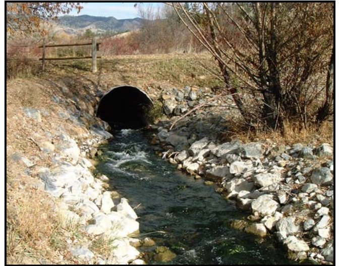
Photo Illustration 1. Upper two photos display a fish passage improvement project on Duck Creek, a tributary to Hebgen Lake. The goal of this project was to improve upstream fish passage, primarily for spawning rainbow trout from Hebgen Lake, through a culvert located on U.S. Highway 191. Photo on left shows perched culvert before project completion. Photo on right shows completion of constructed riffle downstream of culvert. Lower two photos display a fish passage improvement project on Magpie Creek, a tributary to Canyon Ferry Reservoir. The goal of the project was to improve upstream fish passage, primarily for spawning rainbow trout from Canyon Ferry Reservoir, through a culvert located on a U.S. Bureau of Reclamation road. Photo on left shows perched culvert before project completion. Photo on right shows completion of constructed riffle downstream of culvert.
