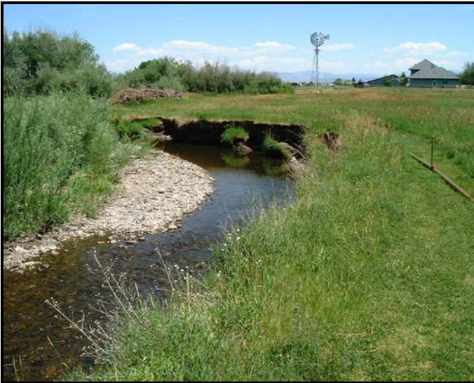
Photo Illustration 7. Upper two photos show a bank stabilization project on the Teton River located near Choteau. The goal of this project was to stabilize an actively eroding stream bank through sloping and re-vegetation and to protect the riparian corridor from livestock over-grazing with fencing. The upper left photo show a portion of the eroding stream bank prior to stabilization. The upper right photo shows the stream bank immediately following treatment. Lower two photos show a bank stabilization project on Tenmile Creek located near Helena. The goal of this project was to stabilize actively eroding stream banks though sloping, rootwads and re-vegetation and to protect the riparian corridor from livestock overgrazing. The lower left photo shows a reach of eroding stream bank prior to treatment. The lower right photo shows the same stream bank after treatment.
