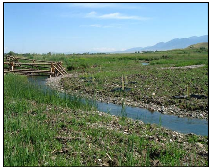
Photo Illustration 6. Top pair of photos shows a channel restoration project on Nelson-Dana Spring Creek, a tributary to the Yellowstone River near Livingston in Park County. The goal of this project was to create spawning and rearing habitat for trout, especially Yellowstone cutthroat trout, and enhance recruitment to the Yellowstone River. Top left photo shows over-widened channel with poor streamside vegetation. Top right photo shows newly restored channel with riparian corridor fencing. Lower pair of photos shows a channel restoration project on Darnutzer Slough, a tributary to the Beaverhead River located south of Twin Bridges in Madison County. The goal of this project was to enhance spawning and rearing habitat for trout and enhance recruitment to the Beaverhead River. Lower left photo shows slough before restoration and lower right photo shows newly restored channel.
