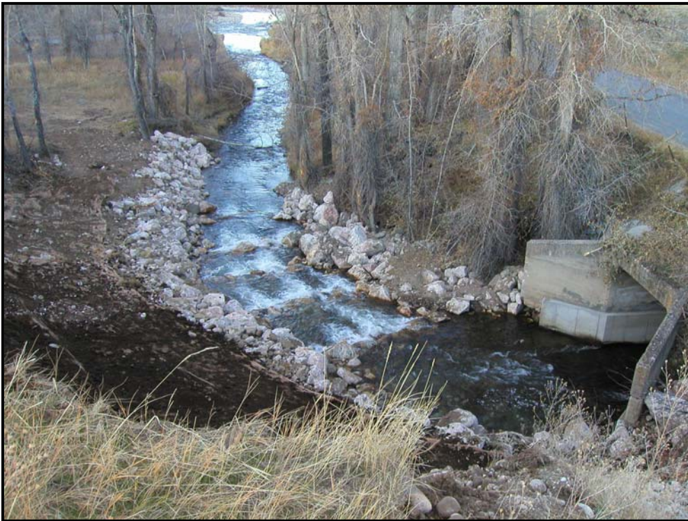
Photo Illustration 2. Fish passage improvement on Clear Creek, a tributary to Rock Creek in Carbon County. The goal of this project was to improve upstream fish passage, primarily for rainbow trout and brown trout, through a box culvert located at a county road near the mouth of the stream. Upper photo shows perched box culvert prior to the project. Lower photo shows the completion of a series of rock stair-step pools downstream from the culvert.
