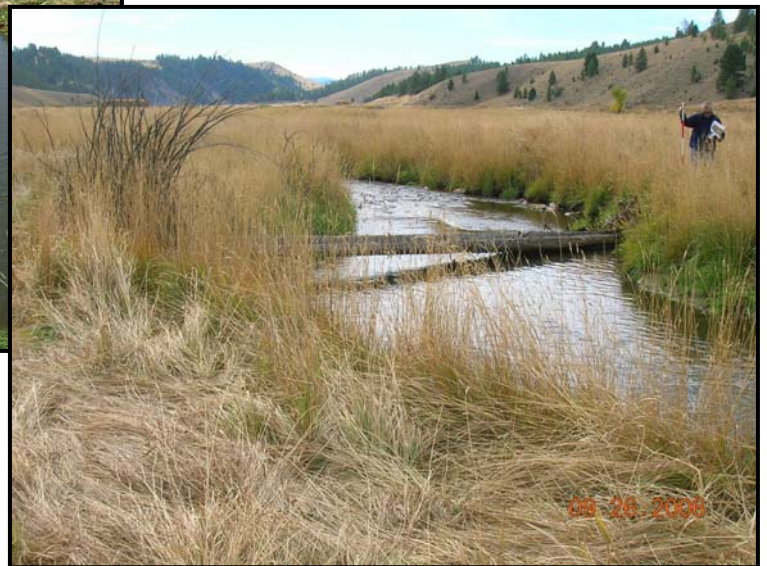
Photo Illustration 4. Restoration of Upper Willow Creek, a tributary to Rock Creek in Granite County. The goal of the project was to restore aquatic habitat and channel function on a 2-mile reach of the stream to benefit westslope cutthroat trout, rainbow trout, brown trout and bull trout. Top photo shows unstable stream channel prior to restoration. Lower left photo shows restored channel two months following channel construction. Lower right photo shows restored channel one year and three months following channel construction.
