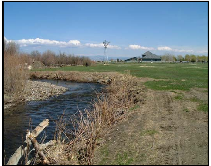
Photo Illustration 7. Upper two photos show a bank stabilization project on the Teton River located near Choteau. The goal of this project was to stabilize an actively eroding stream bank through sloping and re-vegetation and to protect the riparian corridor from livestock over-grazing with fencing. The upper left photo show a portion of the eroding stream bank prior to stabilization. The upper right photo shows the stream bank immediately following treatment. Lower two photos show a bank stabilization project on Tenmile Creek located near Helena. The goal of this project was to stabilize actively eroding stream banks though sloping, rootwads and re-vegetation and to protect the riparian corridor from livestock overgrazing. The lower left photo shows a reach of eroding stream bank prior to treatment. The lower right photo shows the same stream bank after treatment.
