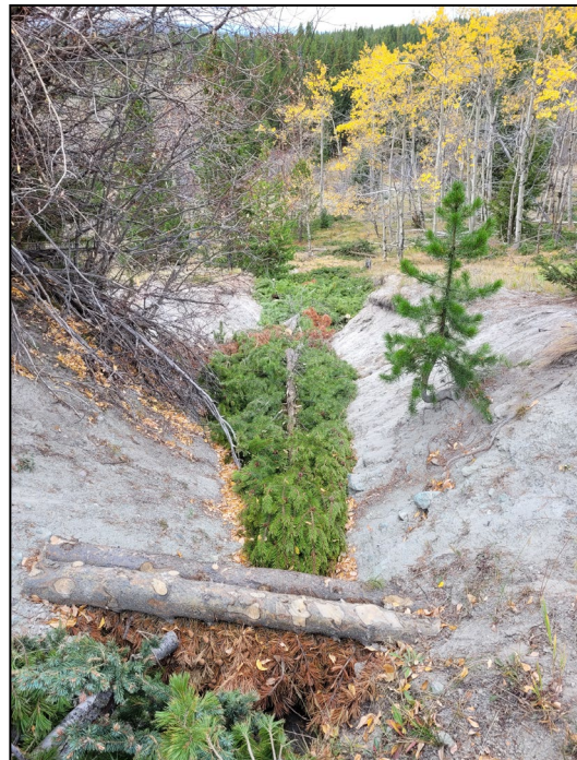
Figure 13 - Cut material from the adjacent aspen stand was placed in this eroded gully to reduce sediment transport into Oregon Creek, October 2022. Image: J. Parke
