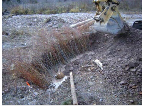
EXAMPLE OF A WILLOW TRENCH INSTALLATION
