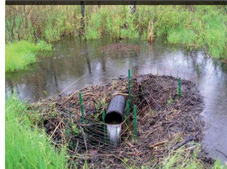
FLOODING SOLUTION Below: Pond-leveling devices like this can lower water levels without having to remove beavers and destroy their dams, which incoming beavers can quickly rebuild in a few days.
