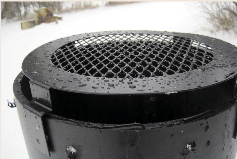
NO ENTRANCE Above: An installed Poo-Poo Screen sits slightly above the exhaust pipe. The design blocks birds while allowing ventilation even if covered in snow. Right: Volunteer Megan Betcher and FWP park maintenance foreman Erik Dion install screens on latrines at Makoshika State Park. FWP has installed screens at state parks and fishing access sites across Montana.
