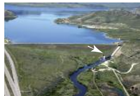
WHERE IT ALL BEGINS Clark Canyon Dam forms Clark Canyon Reservoir south of Dillon (above). Where the dam releases water at its base (arrow) is the start of the Beaverhead River, known for its excellent rainbow and brown trout fishing (right).
