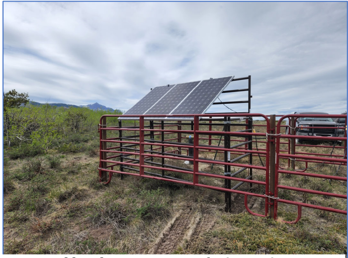
New portable solar pump system for improving livestock grazing distribution and associated wildlife habitat benefits, Blackleaf WMA, June 2022. (Image: R. Rauscher)
