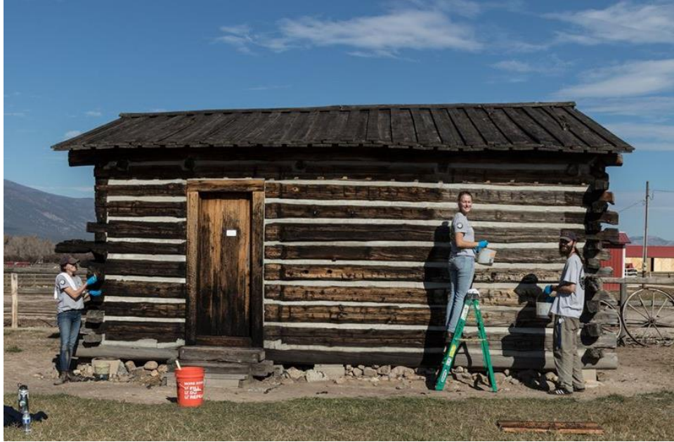
Figure 6: AmeriCorps members help with oiling the wood of the cabin at Fort Owen at a fall 2019 work day organized by the Friends of Fort Owen.
