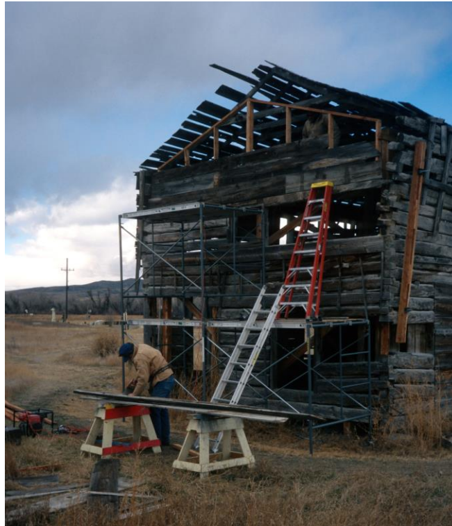
Figure 4: Efforts to stabilize the Gallatin City II Hotel (24GA0355) underway in 2015.
