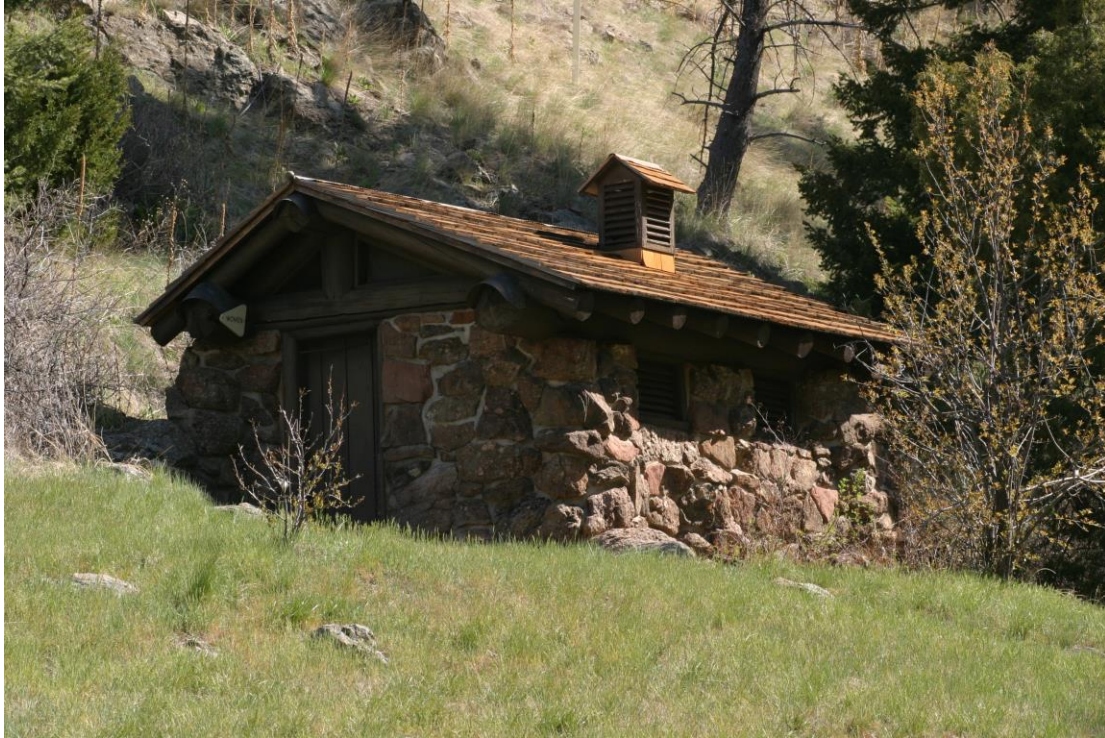
Figure 10: Historic latrine built by the CCC at Lewis and Clark Caverns, now part of the NRHP-listed Historic District.
