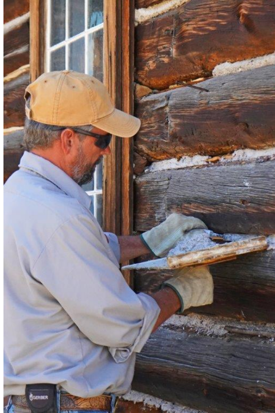
Figure 9: MSP employees working alongside volunteers using historic daubing techniques at the Bannack Institute.
