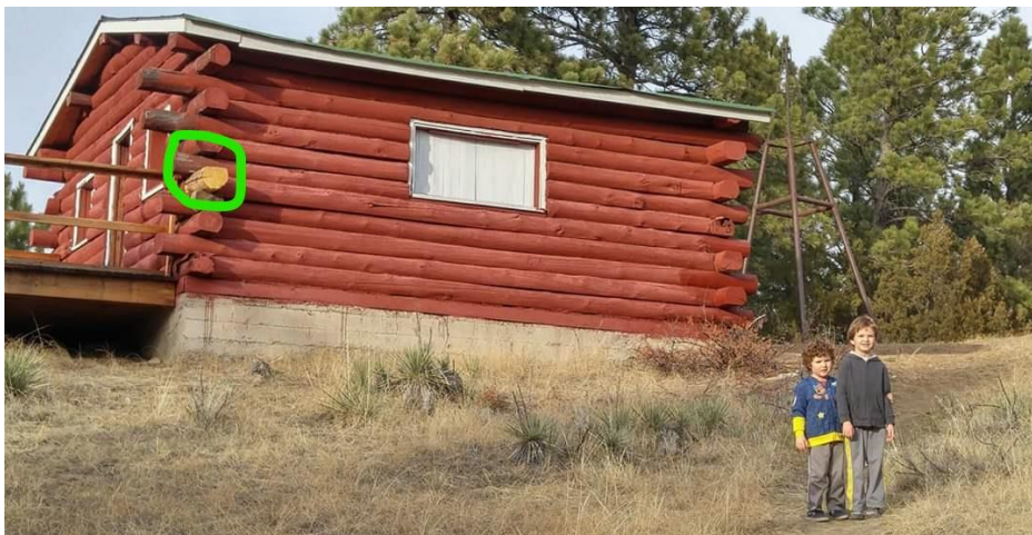
Figure 16: The McCarty Cabin at Makoshika State Park, showing the very last log end to be painted.
