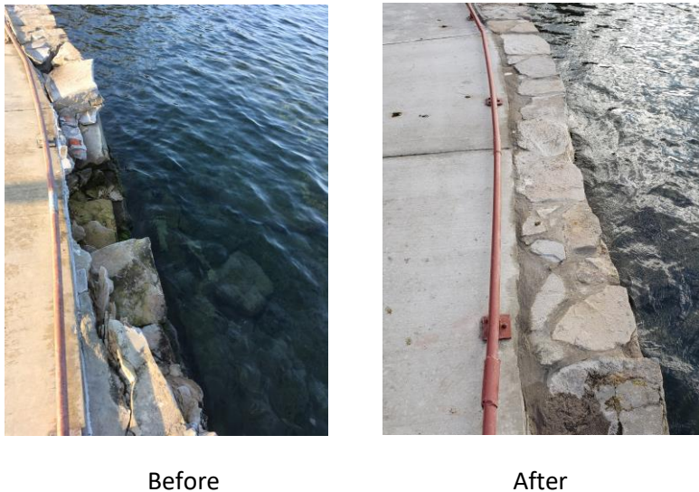
Figure 12: In-kind repairs of historic rockwork on the walkway at Roe Island, Giant Springs State Park.
