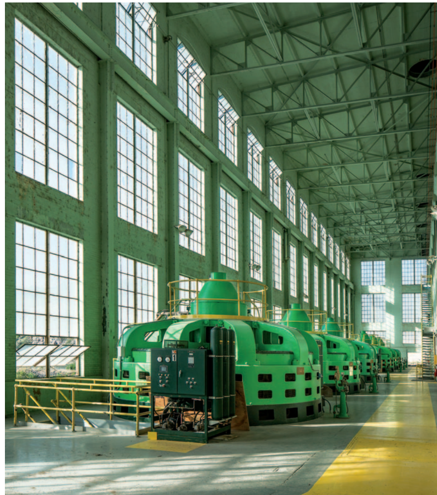
A herd of cattle provides scale to enormous wind turbines, standing 262 feet high, in the Judith Gap Wind Energy Center in central Montana. Below, hydroelectric generators in the powerhouse at Ryan Dam on the Missouri River at Great Falls create energy from the power of water flowing from the upstream impoundment. The five hydropower facilities in and near Great Falls earned it the nickname Electric City.
