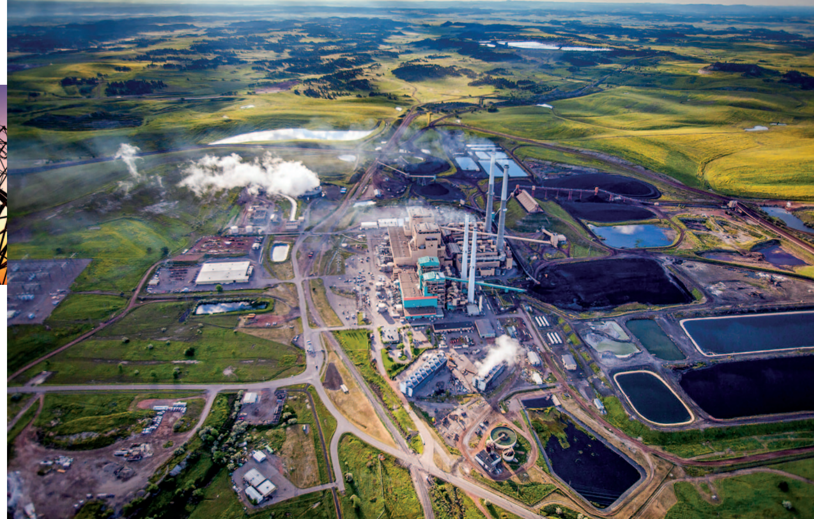
Above: The Colstrip Power Plant, 80 miles east of Billings. Though the plant burns low-sulfur coal and employs state-of-the-art scrubbers to restrict sulfur dioxide emissions to less than levels required by the Clean Air Act, concerns about carbon dioxide and global warming have caused Oregon, a major customer, to scale back purchases of electricity generated by the facility. Below: Montana’s four oil refineries, including this one of two in Billings, refine crude oil mainly from Canada and Wyoming into gasoline, ultra-low-sulfur diesel fuels, aviation fuels, butane, and propane.
