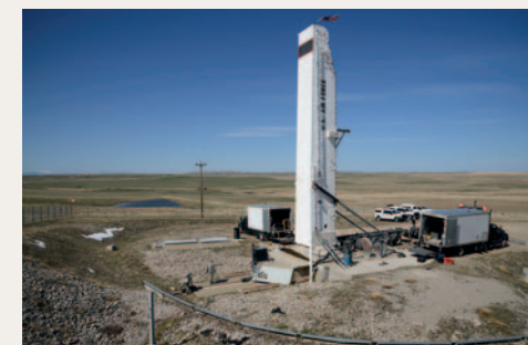
Installing an ICBM silo near Great Falls.
