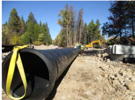
During (siphon pipe)
