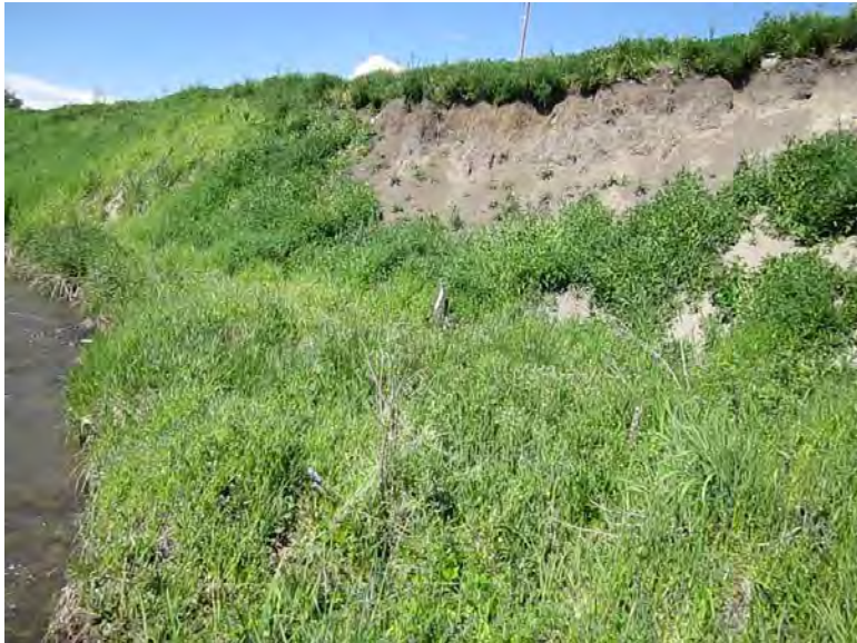
FIGURE 93. FLOODPLAIN BENCH 5 YEARS AFTER CONSTRUCTION.
