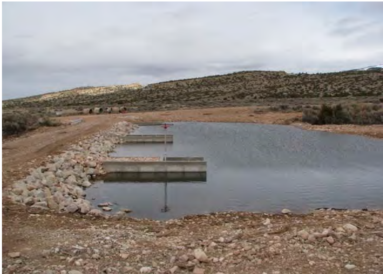
FIGURE 73. STORAGE POND AND GATED STAND PIPES SOON AFTER CONSTRUCTION.
