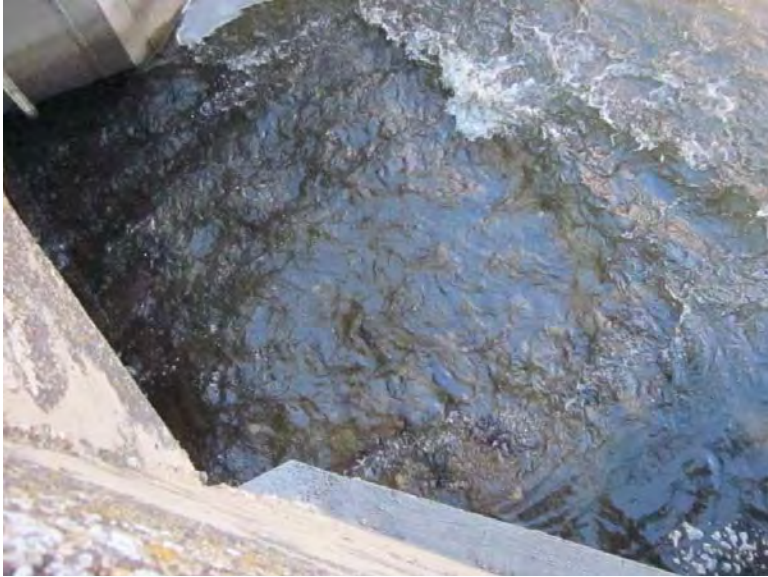
FIGURE 22. OUTLET OF BOX CULVERT ON CLEAR CREEK
