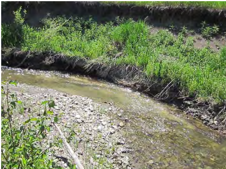
FIGURE 94. CONSTRUCTED FLOODPLAIN BENCH ON SOUTH FORK HORSE CREEK.
