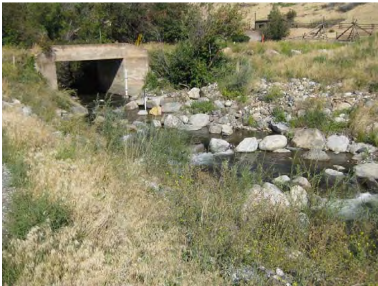
FIGURE 77. STEP-POOL SEQUENCE CONSTRUCTED TO PROVIDE FISH PASSAGE INTO ROCK CREEK.
