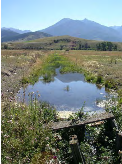
FIGURE 64. PRE-PROJECT PHOTO OF AN EXCAVATED CHANNEL FEEDING THE NELSON/DANA SPRING CREEK.
