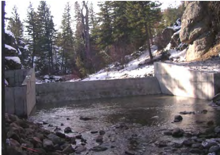
FIGURE 63. NEWLY CONSTRUCTED BARRIER ON LOWER DEER CREEK.
