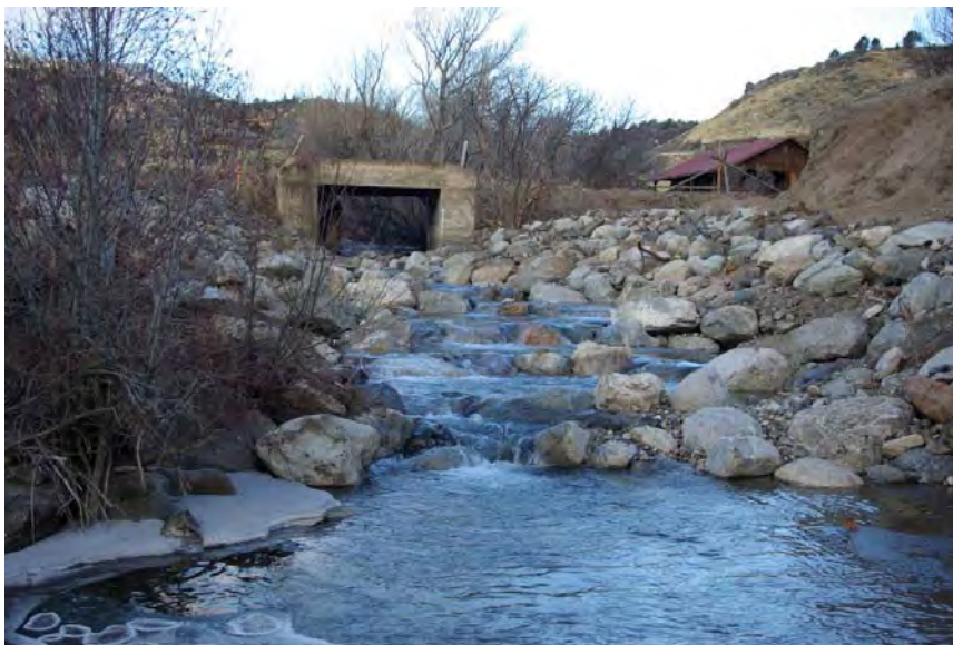
FIGURE 76. NEWLY CONSTRUCTED STEP-POOL SEQUENCE.
