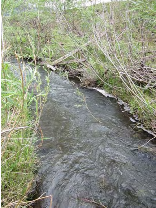
FIGURE 55. EXAMPLE OF CONSTRUCTED RIFFLE, ESTABLISHED WILLOWS, AND UNDERCUT BANKS ON FLESHMAN CREEK.
