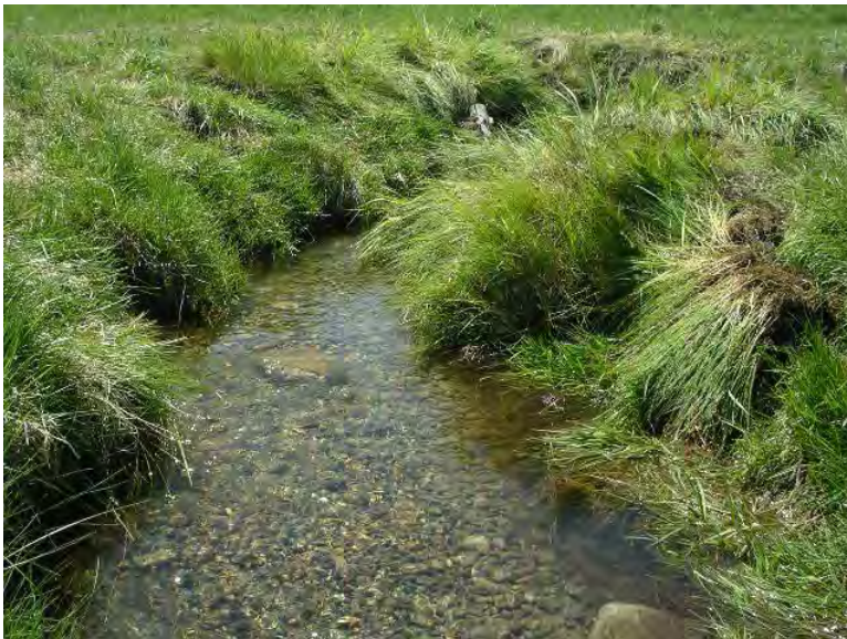
FIGURE 61. RECONSTRUCTED CHANNEL AND IMPORTED SPAWNING GRAVEL.
