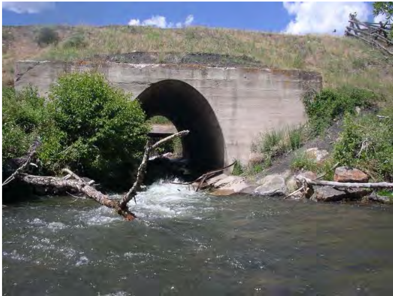
FIGURE 75. RAILROAD CULVERT ON ROCK CREEK.
