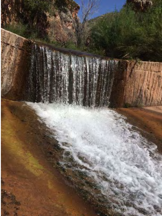
FIGURE 24. SPLASH PAD OF THE CROOKED CREEK BARRIER.
