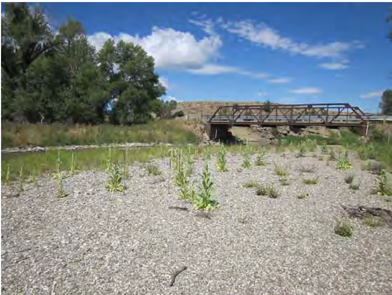
FIGURE 84. EXAMPLE OF LARGE POINT BAR WITHIN PROJECT AREA.
