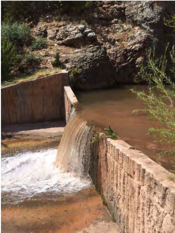
FIGURE 25. VIEW UPSTREAM OF THE FACE OF THE WEIR SHOWING ACCUMULATION OF COHESIVE BED LOAD.
