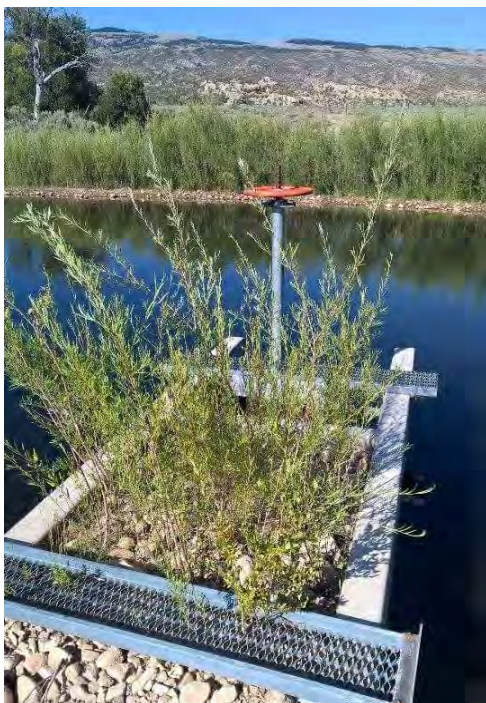
FIGURE 74. STAND PIPE DIVERSION, AND INLET OF PINEY CREEK INTO THE STORAGE POND.
