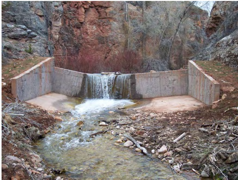
FIGURE 23. NEWLY CONSTRUCTED BARRIER ON CROOKED CREEK, 2008.
