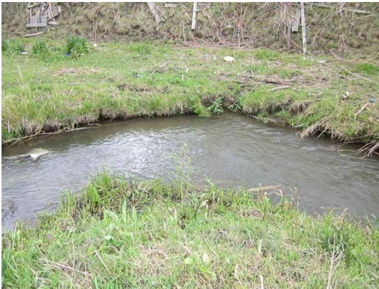
FIGURE 56. OUTER MEANDER BEND SHOWING STABLE BANK CONSTRUCTED WITH COIR FABRIC ENCAPSULATED SOIL LIFTS. (NOTE THAT PHOTO WAS TAKEN IN EARLY JUNE, AND GROUND COVER WAS BEGINNING TO GROW FOR THE SEASON.)
