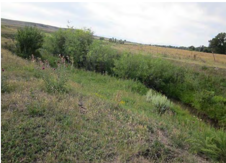
FIGURE 35. EXAMPLE OF REDUCED EROSION AND RECOVERY OF RIPARIAN VEGETATION ALONG A MECHANICALLY SLOPED BANK.
