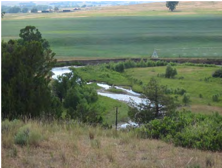
FIGURE 101. AREA OF BANK EROSION ADJACENT TO HAY PASTURE.
