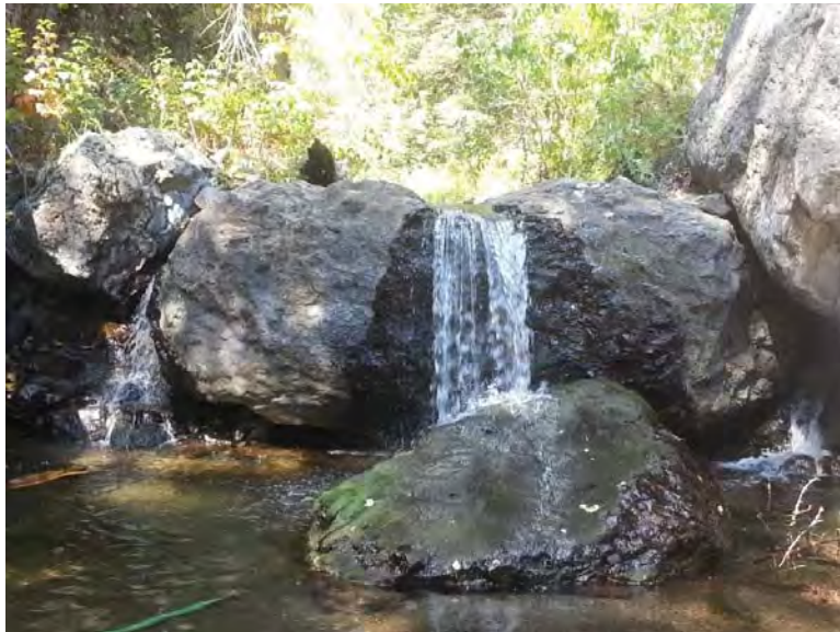
FIGURE 8. BAD CANYON BARRIER AFTER REPAIR AND MAINTENANCE.
