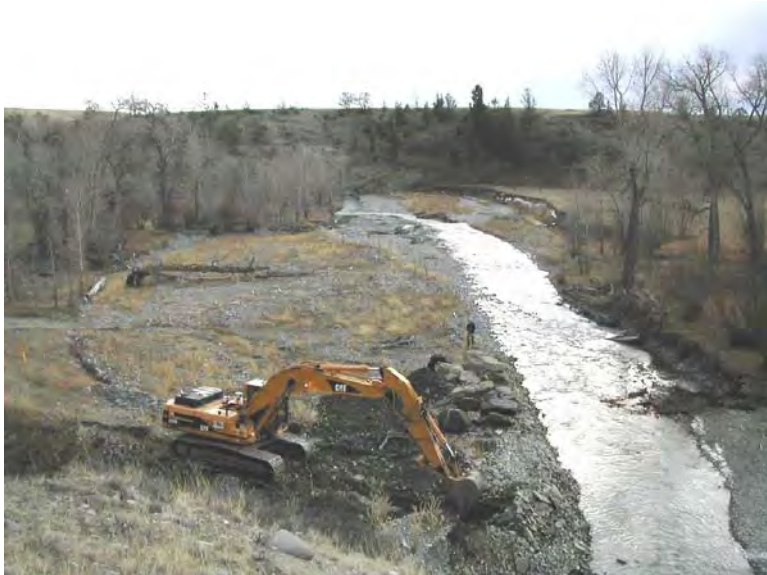
FIGURE 9. CHANNELIZED REACH OF BIG TIMBER CREEK.
