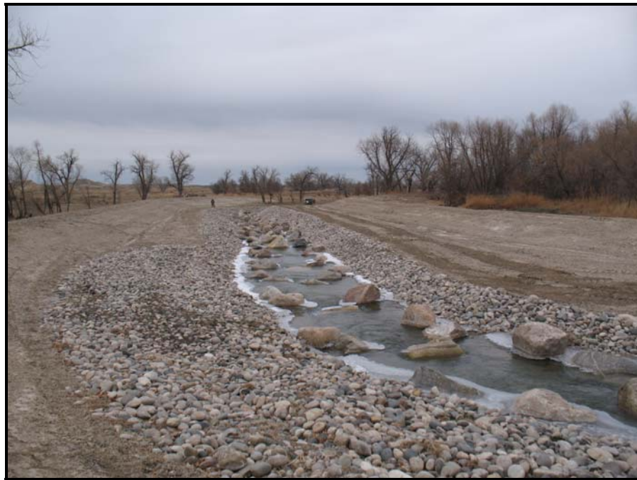
Photo Illustration 5. Upstream fish passage at the T&Y diversion on the Tongue River, a tributary to the Yellowstone River near Miles City. The T&Y diversion dam, located about 20 miles upstream from the confluence with the Yellowstone River, acted as a fish passage barrier and blocked spawning runs of fish from the Yellowstone and lower Tongue. A fish passageway was constructed around the diversion, enhancing upstream passage for a rich assemblage of native warm water fishes. The upper photo shows construction activity on the passageway with the dam showing on the extreme right. The lower photo shows the completed passage channel.
