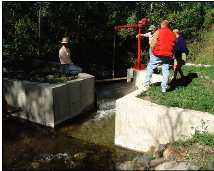
Photo Illustration 4. Fish screens installed on two irrigation diversions to prevent fish from being lost down irrigation systems and, at the same time, allowed water users to obtain their water in an unimpeded manner. The upper photo shows a coanda style fish screen and fish passage ladder installed on Murphy Spring Creek, a tributary to the North Fork Blackfoot River. The stream is important to both westslope cutthroat trout and bull trout. The lower photo shows a drum style screen installed in a diversion located on Big Creek, a tributary to the upper Yellowstone River. Big Creek supports significant spawning runs of Yellowstone cutthroat trout.
