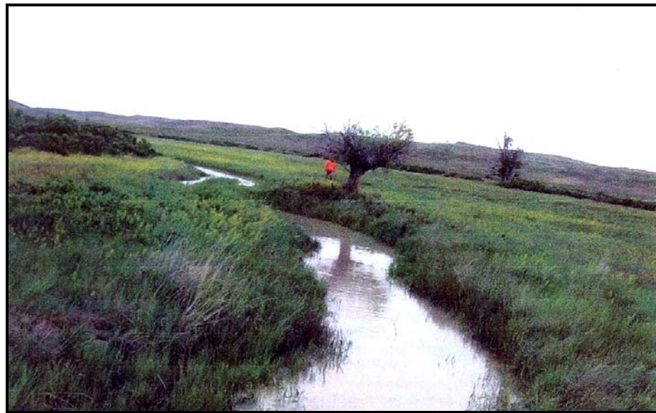
Photo Illustration 7. Channel restoration on Box Elder Creek, a tributary to Telegraph Creek and ultimately Fort Peck Lake. The project restored watershed connectivity by reconstructing a natural meandering channel that historically had been leveled for farming practices. The project also is working towards re-establishing native prairie grasses and streamside woody vegetation. The upper photo shows the area where the stream channel had been obliterated by past farming practices. The lower photo shows the newly restored channel. This project benefits a diverse assemblage of native prairie fish species.
