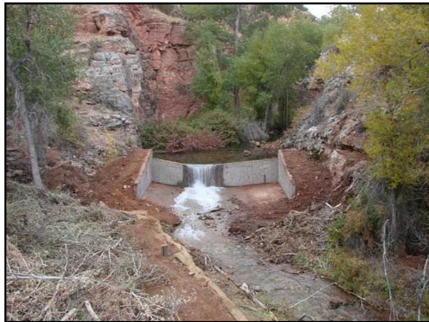
Photo Illustration 2. Fish passage barrier construction on Crooked Creek, a tributary to the Big Horn River, located south of Billings. Crooked Creek supports one of the eastern most populations of Yellowstone cutthroat trout. A natural passage barrier that protected the genetic integrity of the population washed out during a 100-year rainstorm. This project involved reconstruction of a passage barrier near a natural bedrock constriction to protect this unique population from invasion by non-native fishes. The upper photo shows the barrier under construction and the lower photo shows the barrier upon completion.
